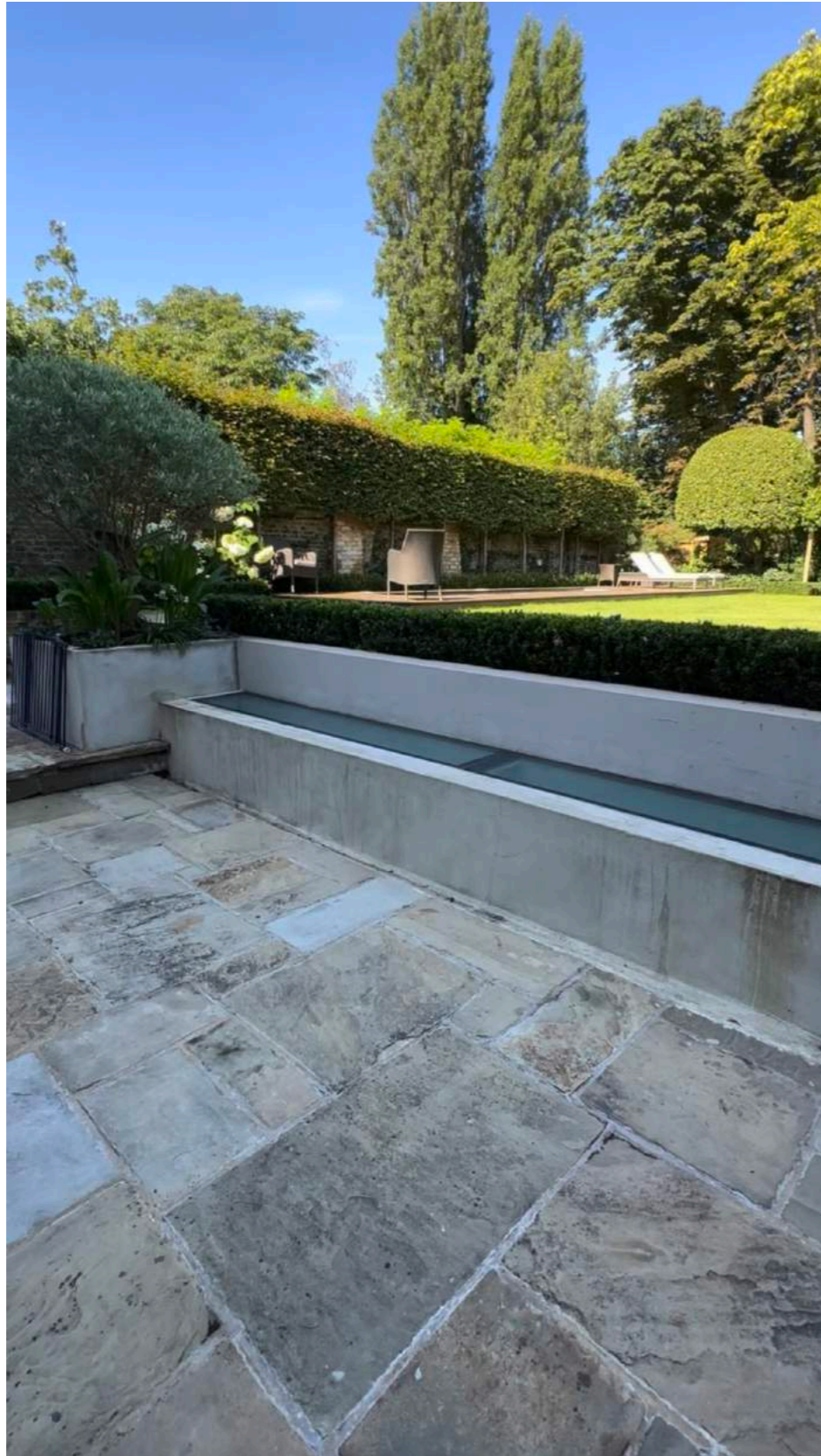
View of the existing rooflight to basement roof
