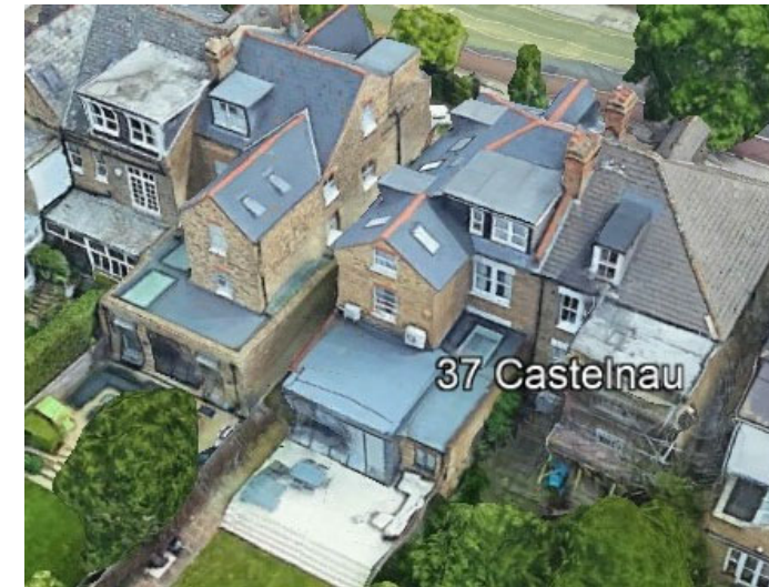
Figure 12 Similar development at 37 Castelnau showing part 1, part two storey rear extension and a full width dormer extension
