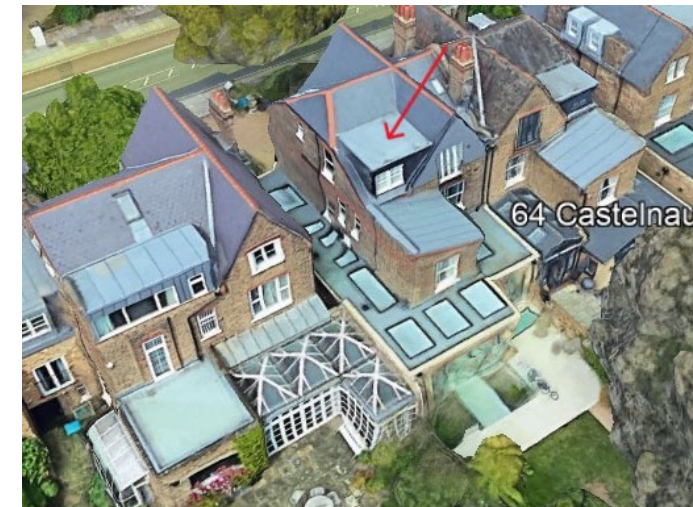
Figure 13 Similar development at 64 Castelnau showing part 1, part two storey rear extension and a full width dormer extension
