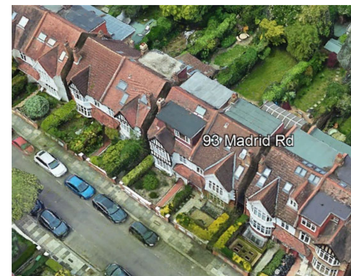
Figure 14 Figure 14 Similar development at 93 Madrid Road Castelnau showing a full width Dormer extension at front and rear
