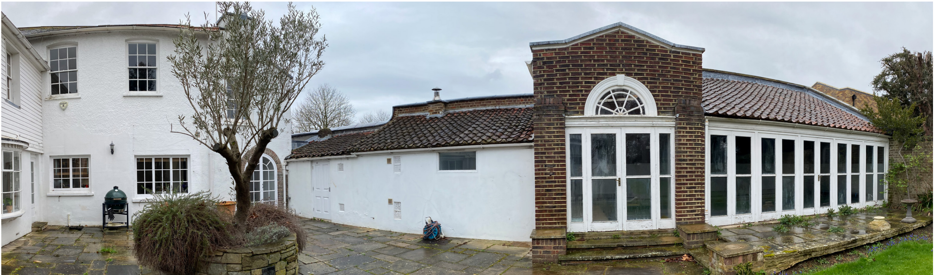
Courtyard view looking north west
