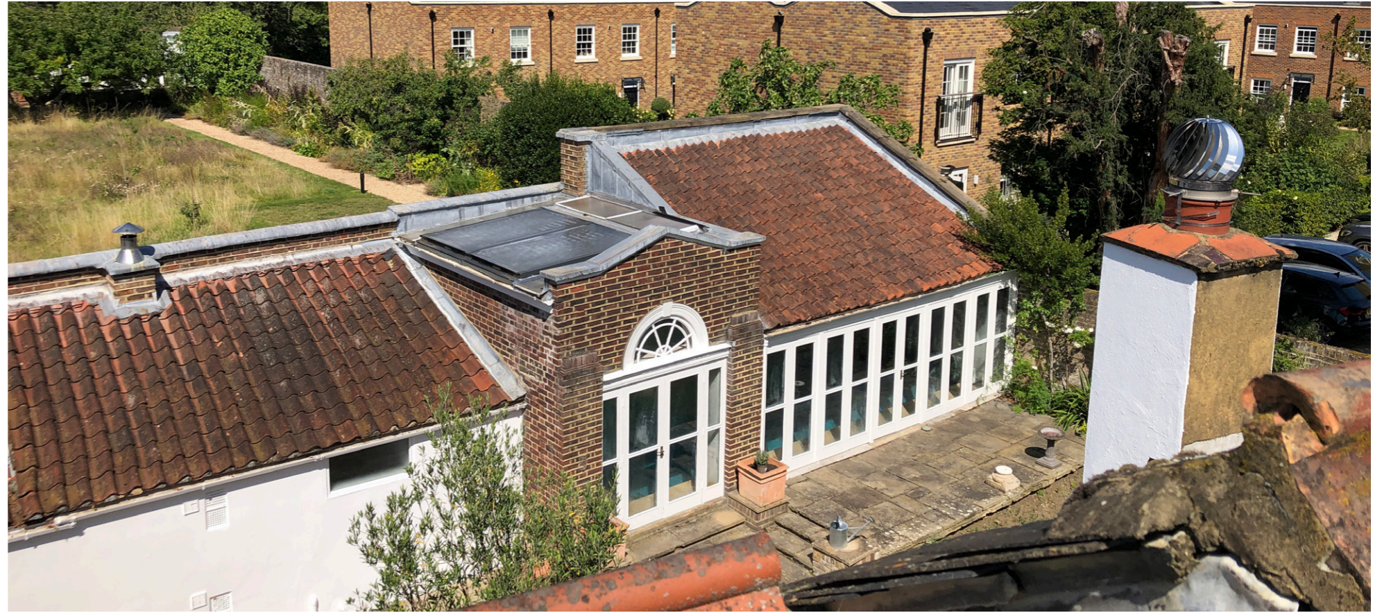
View of pool wing from main house roof
