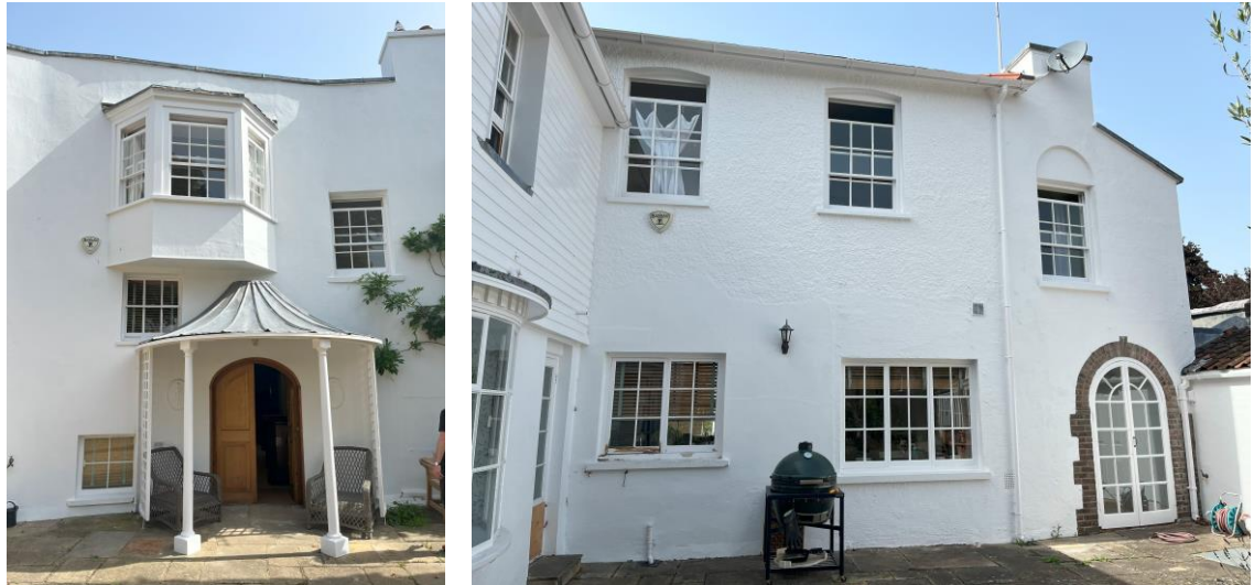
Figures 26 and 27: Main entrance (left) and rear elevation (right) showing some of the later alterations and additions to Avenue Lodge
