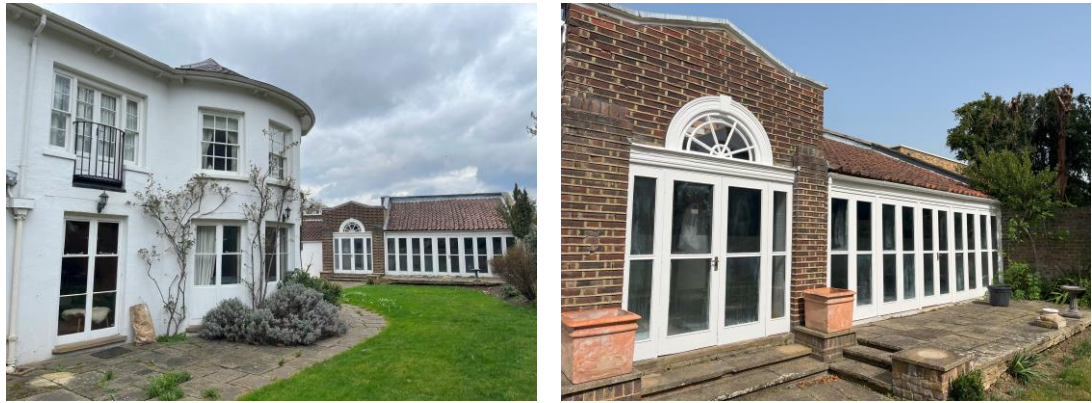
Figures 20 and 21: Ancillary range to the north of Avenue Lodge
