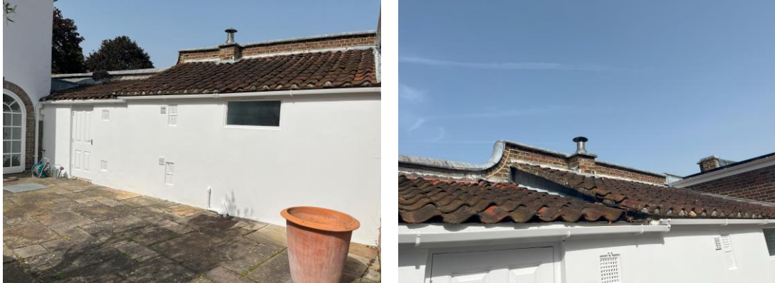
Figures 16 and 17 Ancillary range to the north of Avenue Lodge
