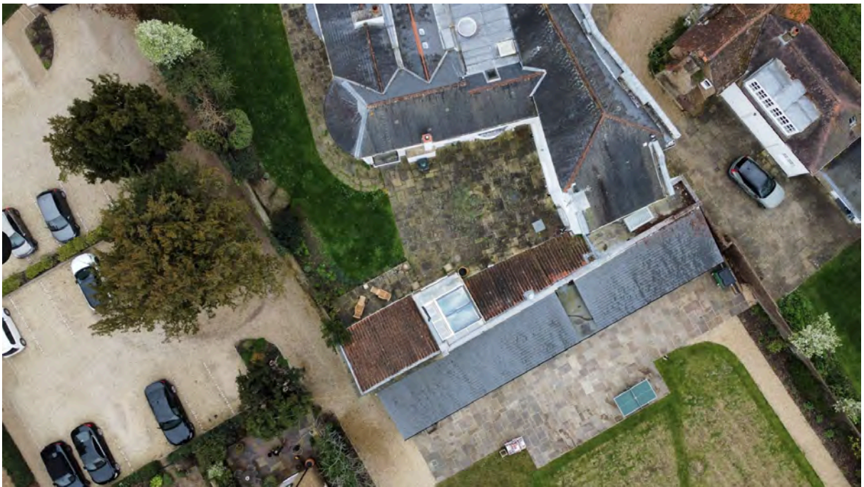
Photographic plate showing the existing pool house layout. (ROAVR GROUP, 2024)
