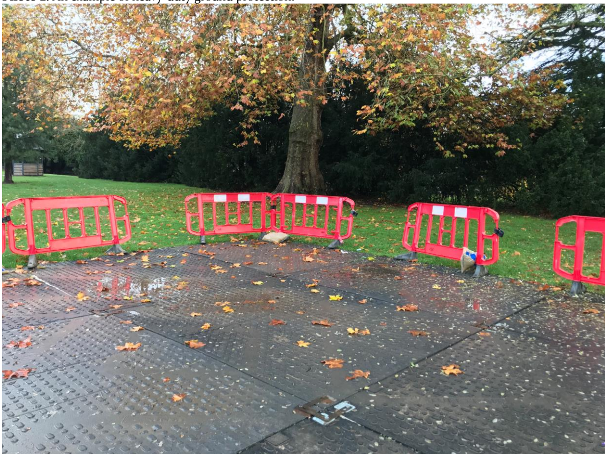
Photo 2. An example of heavy-duty ground protection.
