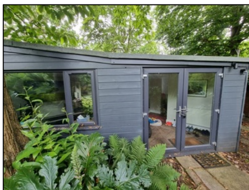
Figure 17 – northern elevation of the outbuilding
