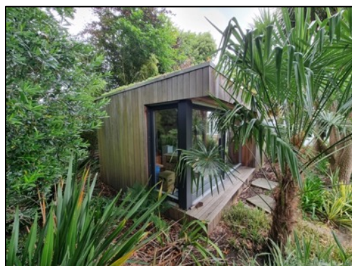
Figure 15 – south-eastern corner of the outbuilding
