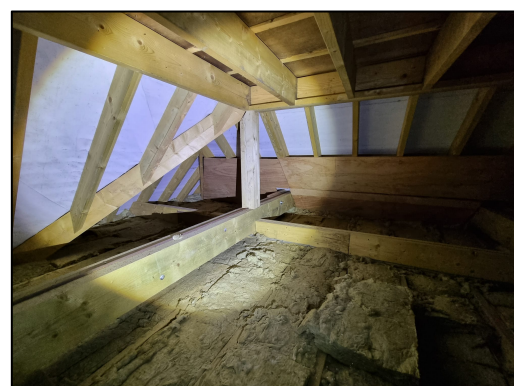
Figure 11 – half-height roof void inside the hipped extension
