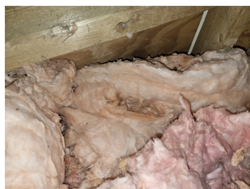
Figure 18 – fibreglass insulation infilling the void space
