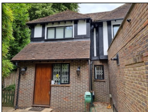
Figure 10 – western hipped extension
