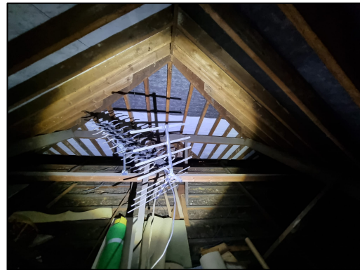
Figure 8 – interior roof void looking southeast
