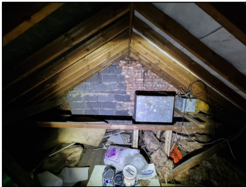
Figure 7 – interior roof void looking northwest
