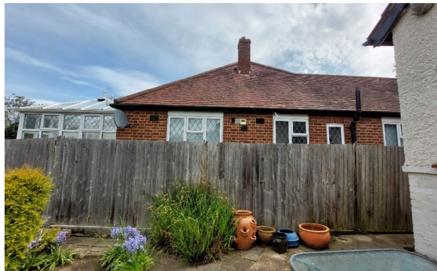
Side of no.101 Atbara Road
