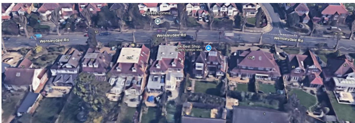
Fig 9 – The west side of Wensleydale Road, development pattern
