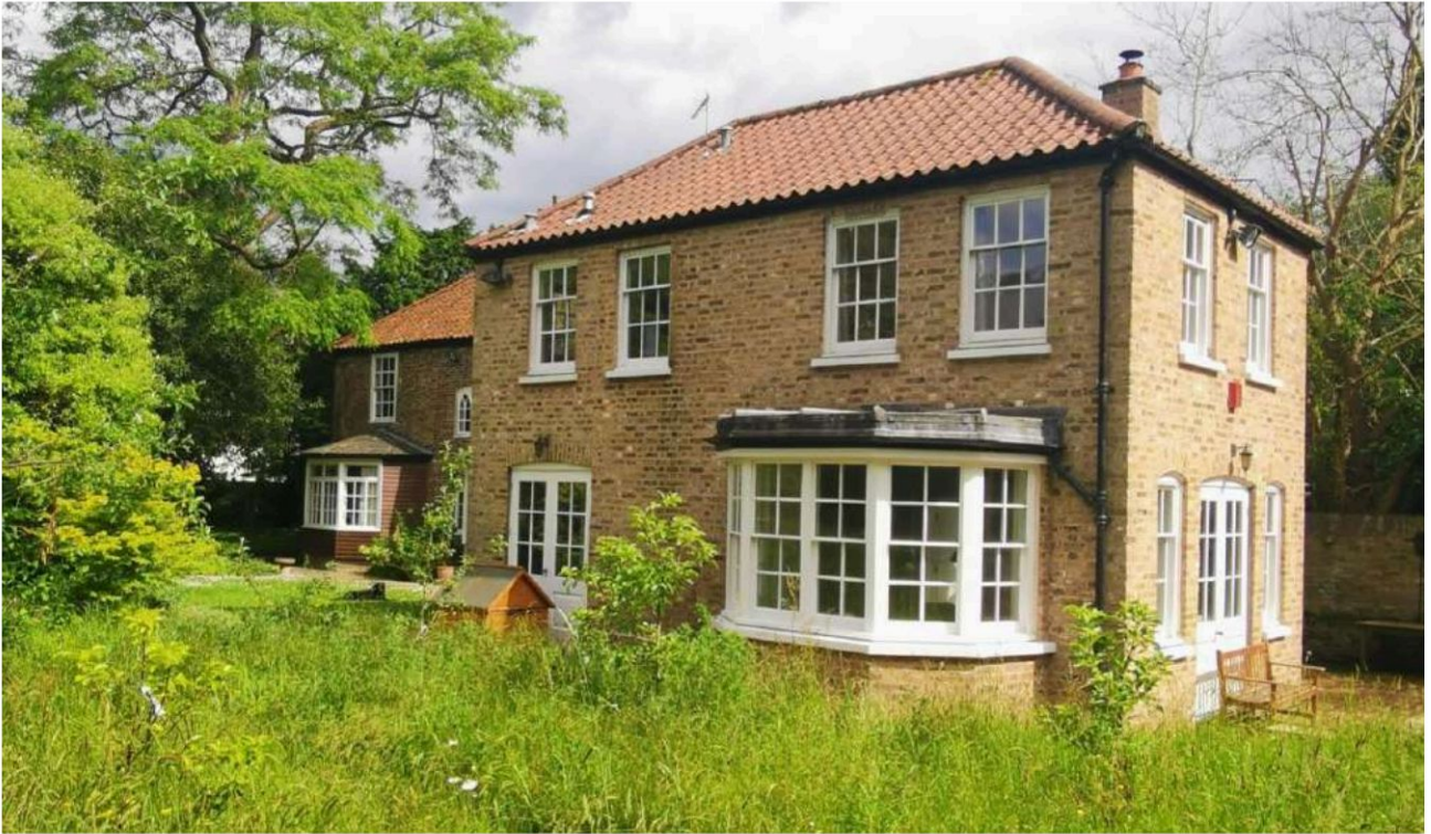
Fig 21: View of the two-storey extension created in the 90s with the 17C wing in the background
