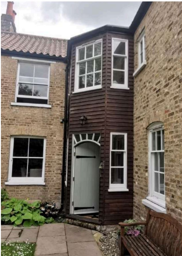
Fig 53: Existing entrance bay structure
