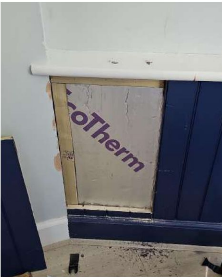
Fig 17, 18: Removal of the modern panelling and timber cladding in the bays exposes modern buildups behind.
