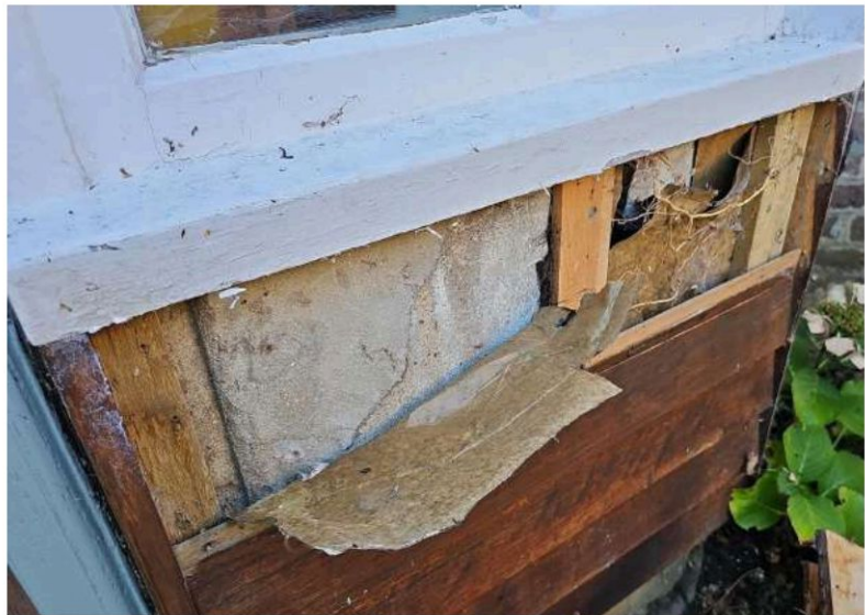
Fig 17, 18: Removal of the modern panelling and timber cladding in the bays exposes modern buildups behind.
