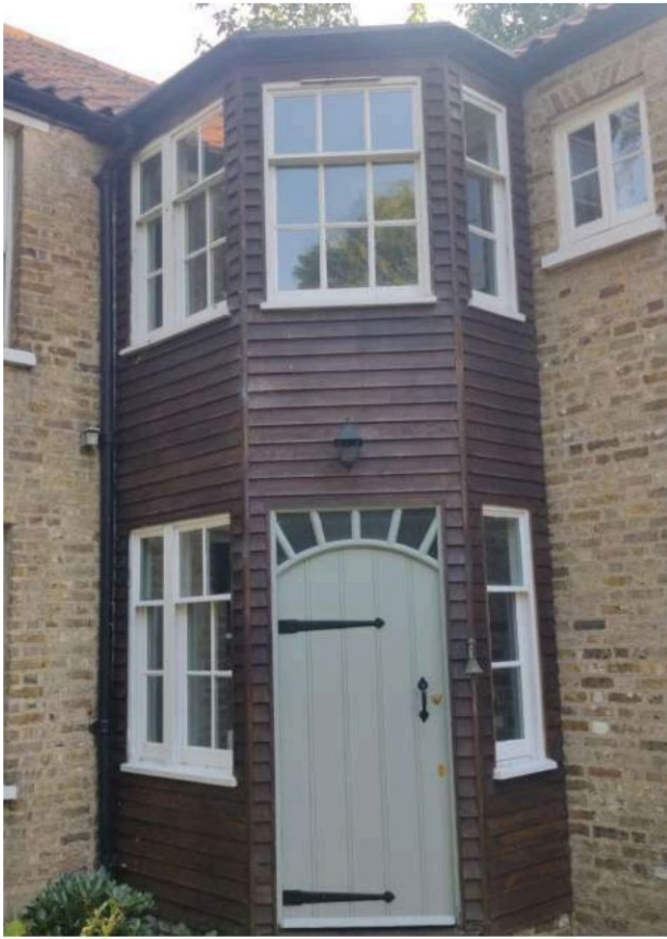
Fig 51: Existing entrance bay structure
