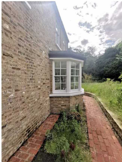
Existing Paving to North Elevation Dining Room Bay
