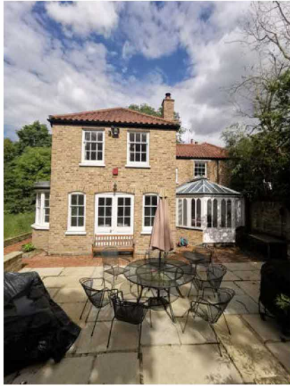
Existing paving to patio area
