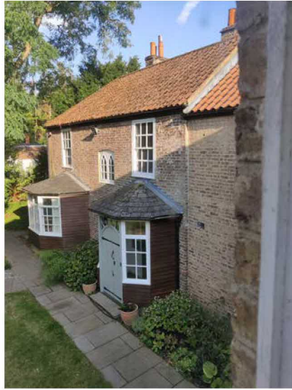
Existing paving to North Elevation
