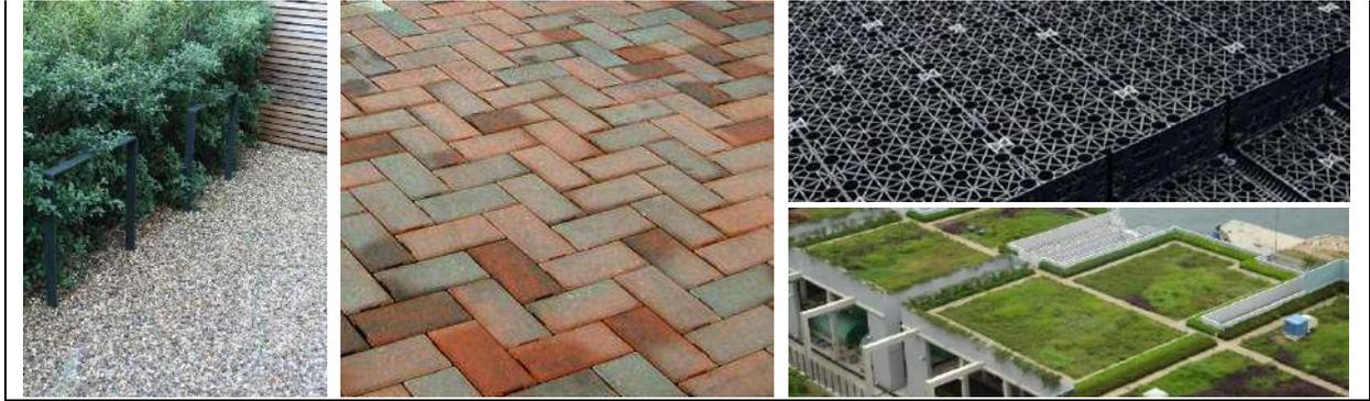
**Figure 3:** Surface water storage facilities and potential SuDS features - rainwater harvesting, on-site tank storage, rain garden soak-away and green roofs. (Source: UK SuDS Manual)
