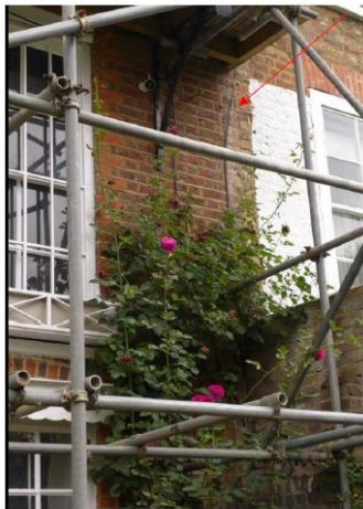
Pl.6: Evidence of once taller garden wall between No.59 and 61.
