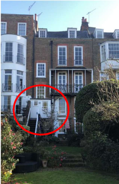
Image of the rear of the dwelling, red circle 1 around the existing to be removed rear element
