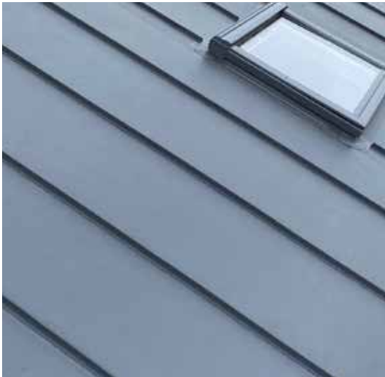
6. Single ply waterproof membrane Single ply roofing membrane with the appearance of a standing seam roof.
