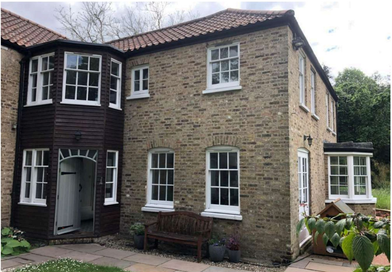
Fig 20: View of the two-storey extension created in the 80s with the side entrance timber structure to the left added in the early 2000s.
