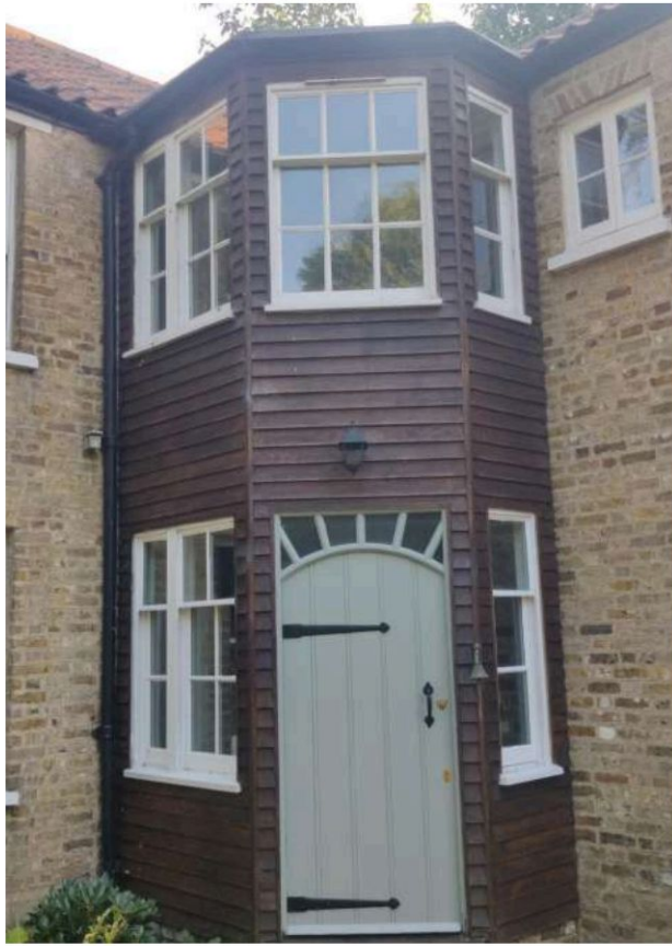
Fig 51: Existing entrance bay structure
