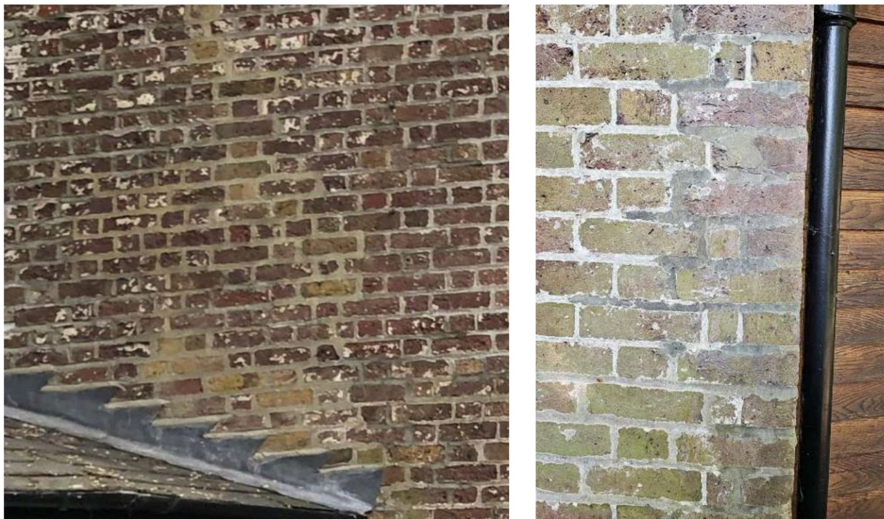
Fig. 23, 24 : Note the use of modern cement pointing on the 17C wing.
