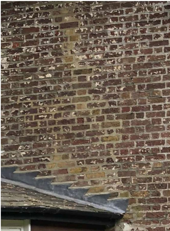
Fig 59: Cement pointing repairs on 17C wing.
