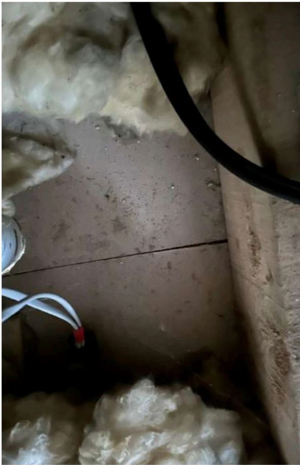
Fig 39, 40: The ceiling of the hall to the 90s wing is clearly modern with use of modern timber, chipboard, insulation and plasterboard.
