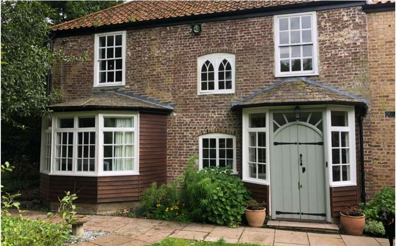
Fig 06: 17C part of the house The modern timber bays were constructed in the 1970s..
