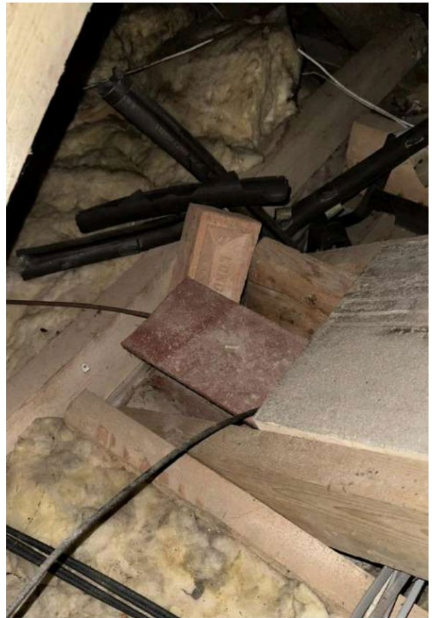
Fig 39, 40: The ceiling of the hall to the 90s wing is clearly modern with use of modern timber, chipboard, insulation and plasterboard.
