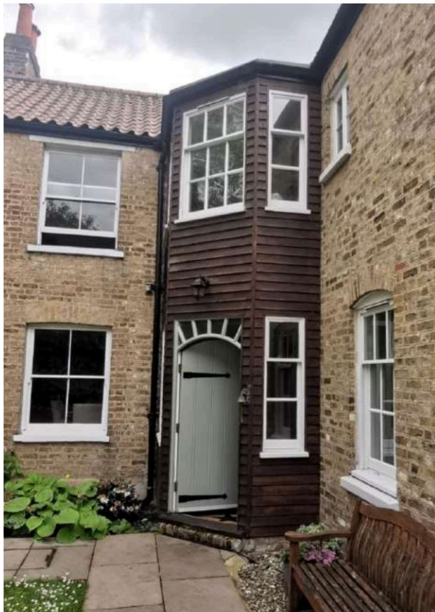
Fig 53: Existing entrance bay structure
