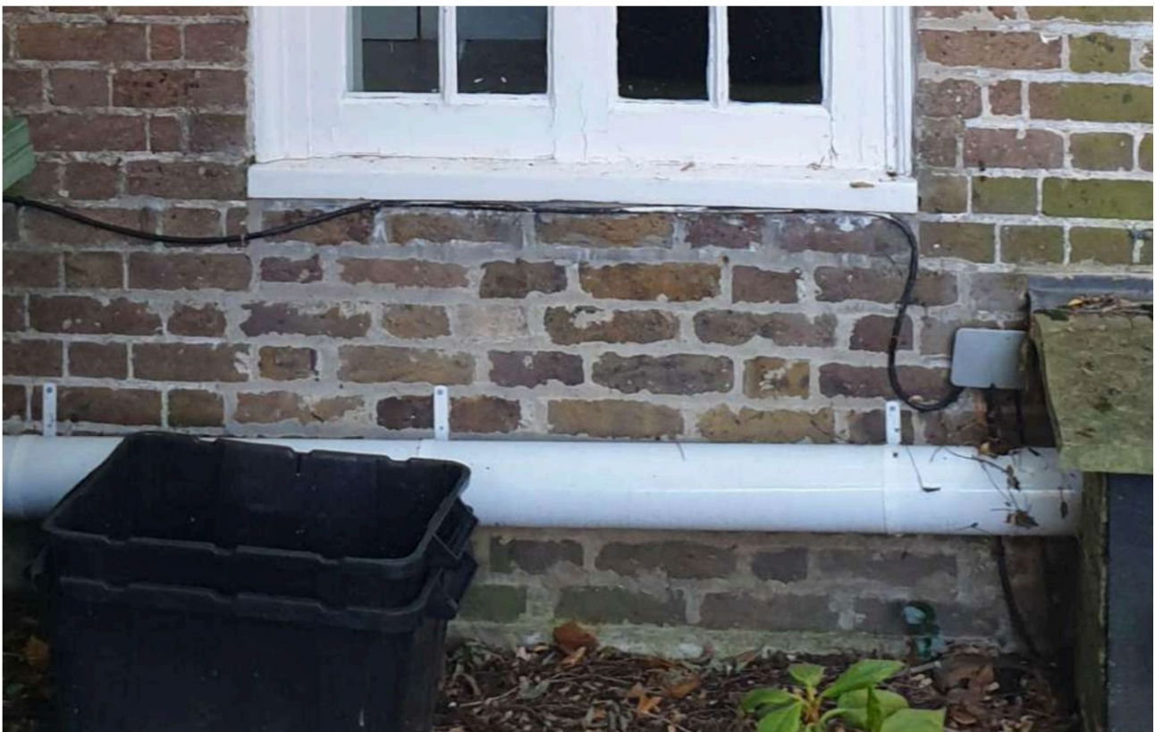
Fig 11: Image of brickwork below window on front elevation showing infill brickwork from earlier entrance door.
