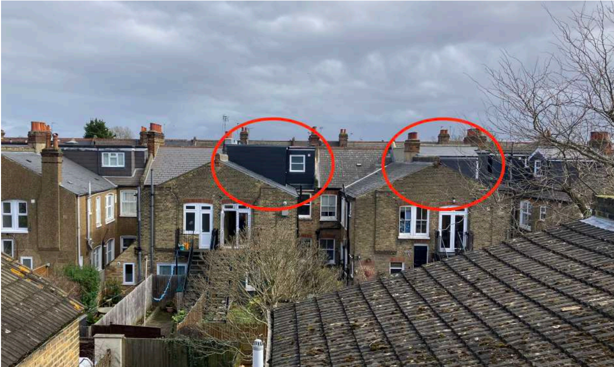
Figure 6: View over outrigger roof (with 54 Ashleigh Road's dormer beyond).
