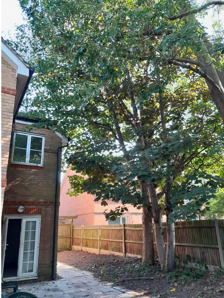
Figure 4 – T1 & T2: Encroaching onto house
