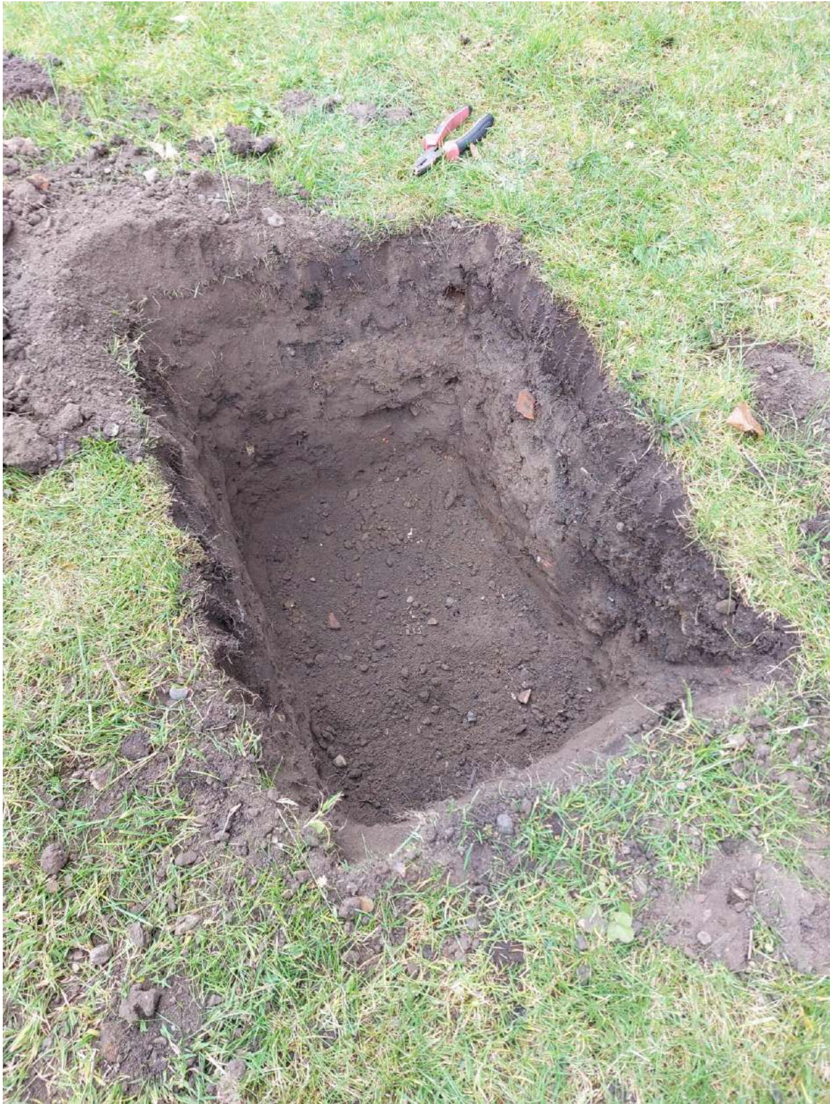
Showing trial pit dug in approximate location marked on Tree Protection Plan, where proposed elevation of new building intersects edge of tree T3's RPA. No roots encountered when digging pit, or visible in edges/base.
