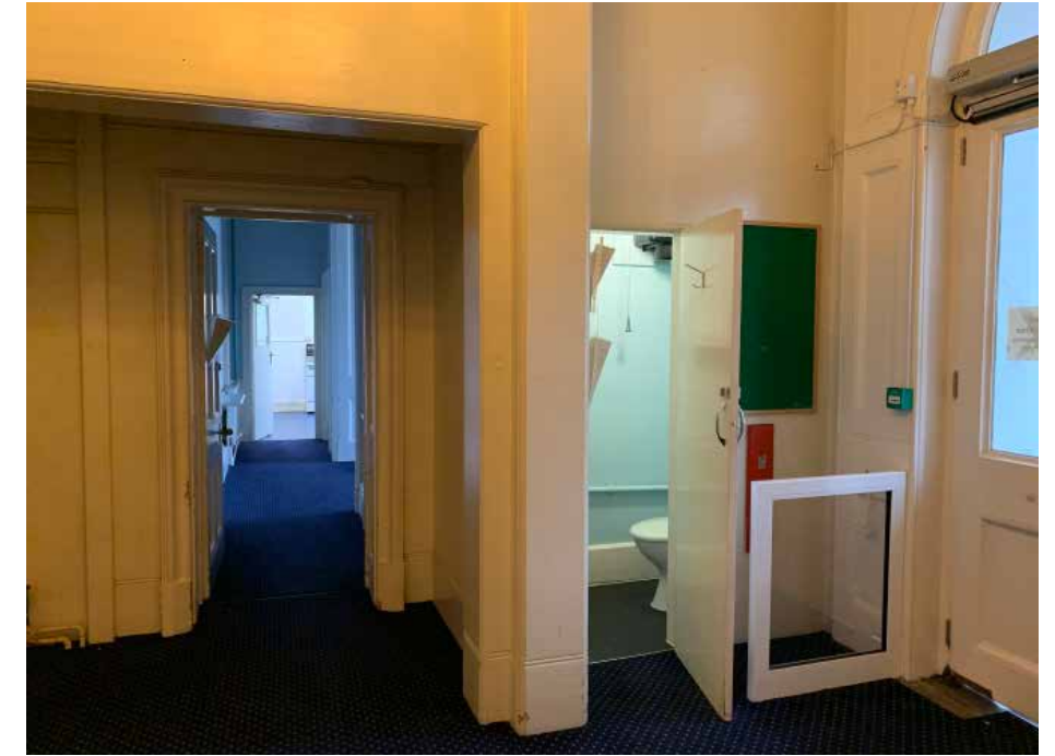
Figure 4.16 The plan of the rear entrance hall has been much altered by the blocking up and creation of new openings.
