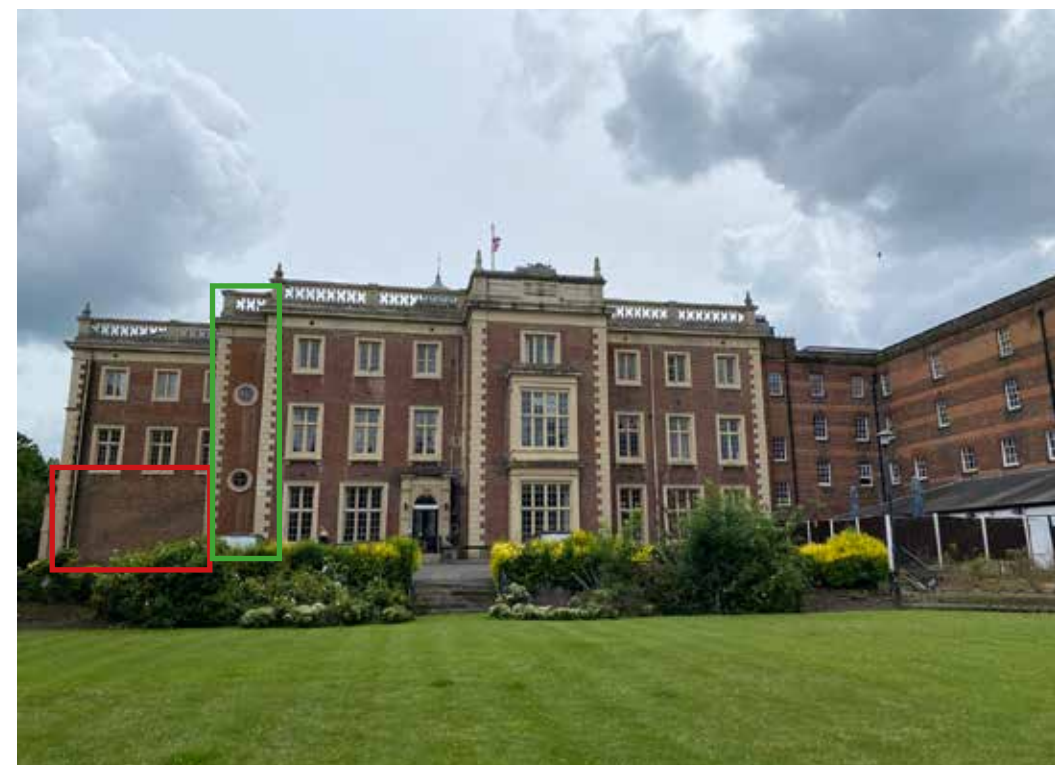
Figure 4.2 Rear north elevation of the hall. Red = exposed brickwork belonging to Hardwick's nineteenth-century wing. Discolouration in the brickwork indicates the location of a former staircase and terrace in this location. Green = a 1970s staircase tower which responds well to the architectural treatment of the hall's exterior.
