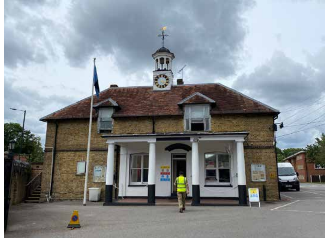
Figure 4.29 The Guardroom, located west of the hall
