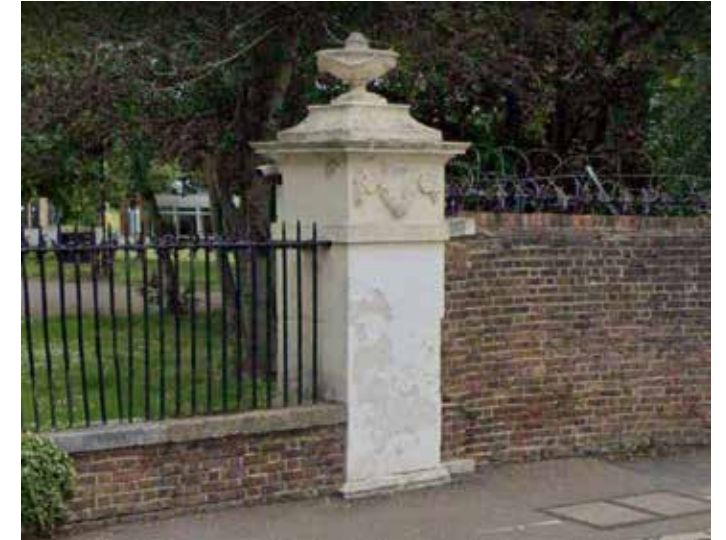
Figure 3.44 Photograph of a stone gate pier which marks the junction between the boundary wall and boundary railings
