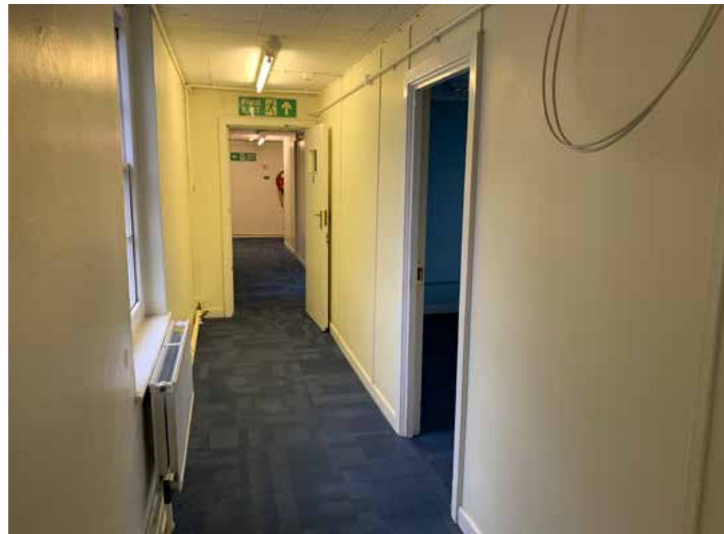
Figure 4.26 Modern partition walls have been introduced into the west wing to create corridors
