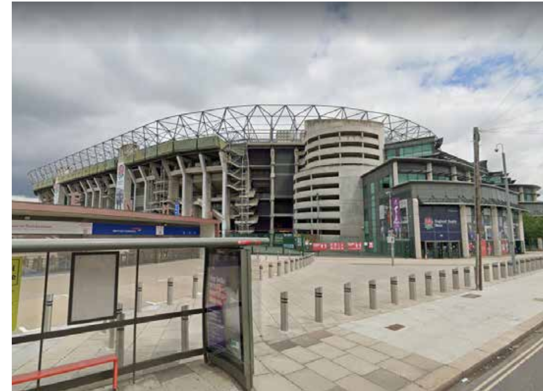
Figure 4.38 The Twickenham Stadium complex is located east of the Site Google Streetview
