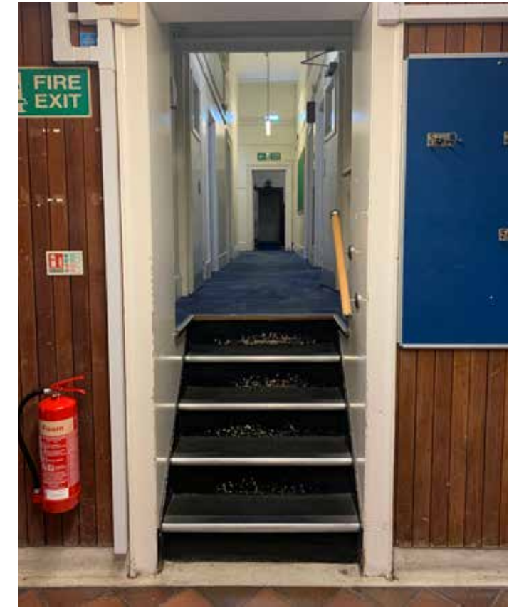
Figure 4.20 A set of steps connecting the 1970s staircase and adjacent corridor is considered to detract from the significance of the building
