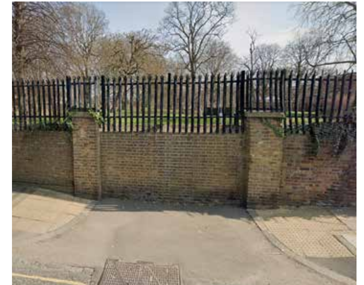
Figure 5.3 Photograph of the existing blocked gate entrance on the west boundary wall of the Site
