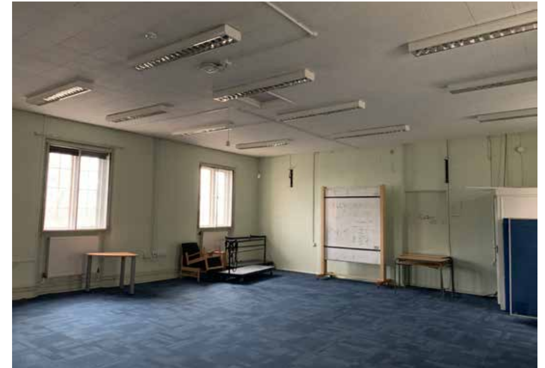
Figure 4.23 A modern dropped ceiling, window grilles, carpet and electrical fixtures have been installed in a front classroom at second-floor level
