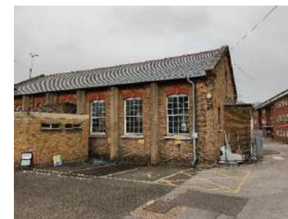
Photo 5 Remedial piers formed of encased steels (back-to-back channels) which anchor remedial ties to the trusses in the Bank Practice Hall
