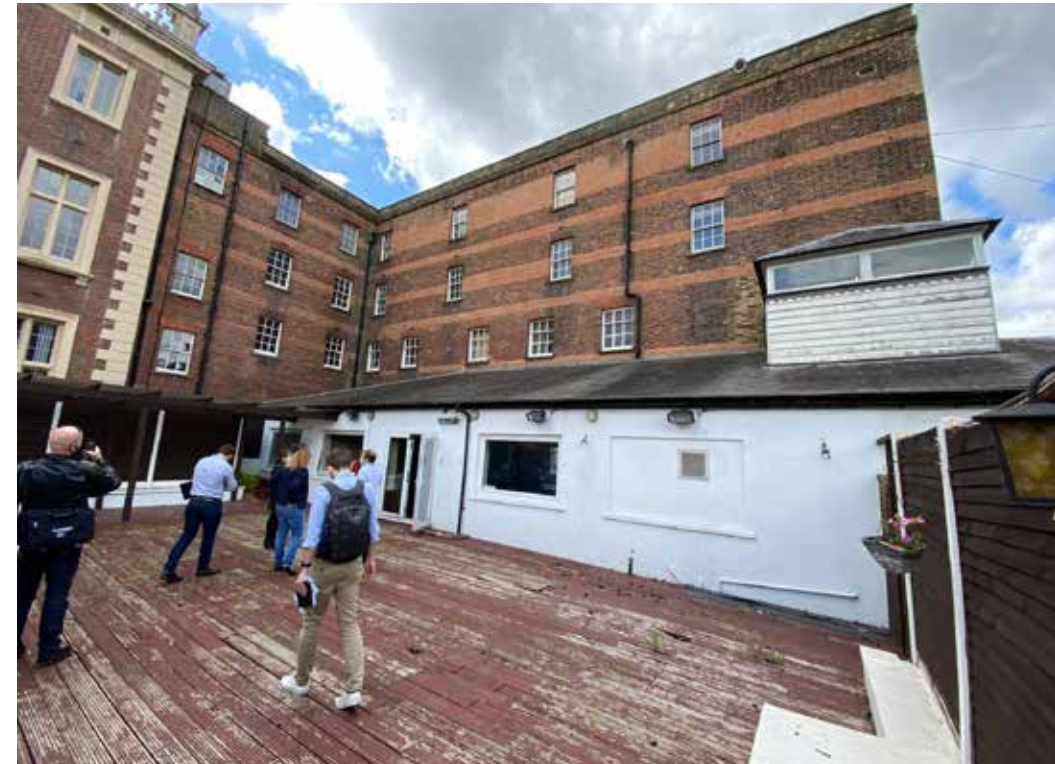
Figure 4.3 Rear north elevation of the hall, showing the new central range designed by George Mair (left) and the early-nineteenth century service wing (right). The rebuilt 'covered way' is shown in the foreground and the twentieth-century staircase tower is also visible.
