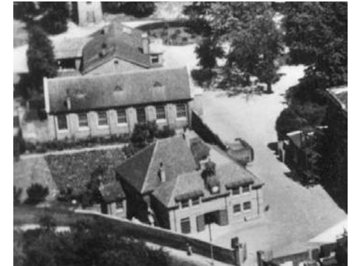
Figure 3.39 Detail of the 1935 aerial photograph of the Site, showing the Guard House (foreground) and Band Practice Hall (background).
