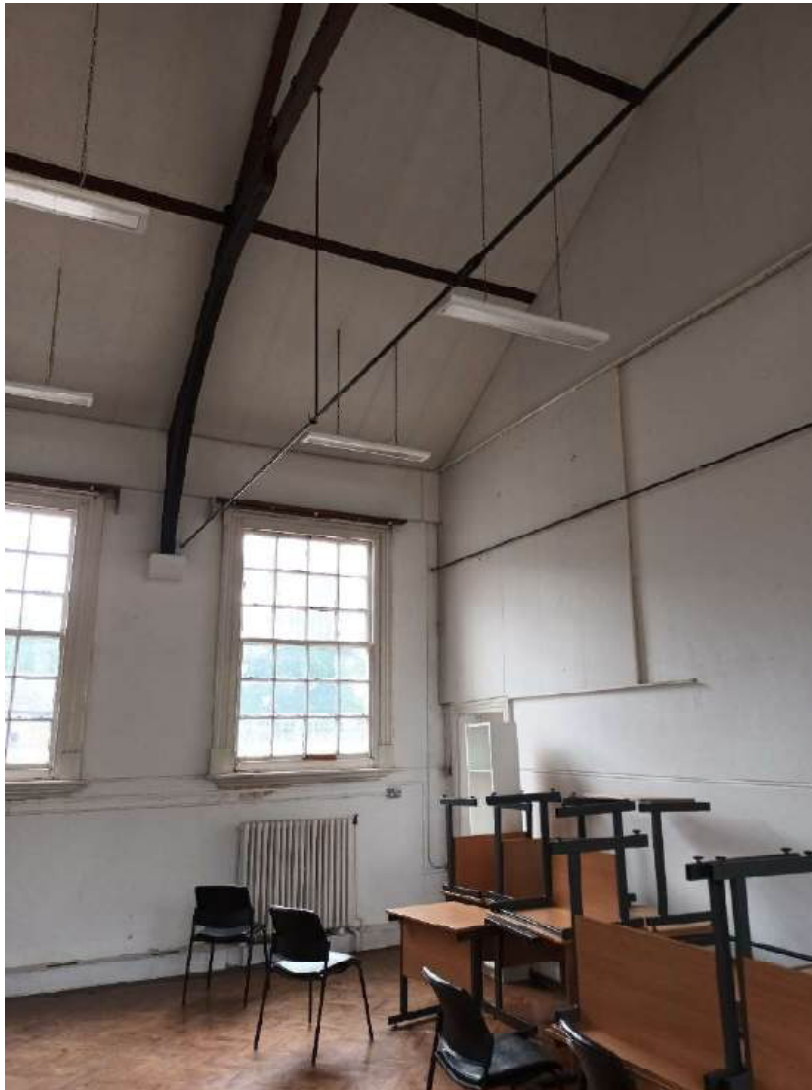
Photograph taken inside the Band Practice Hall, looking towards the internal wall to be removed
