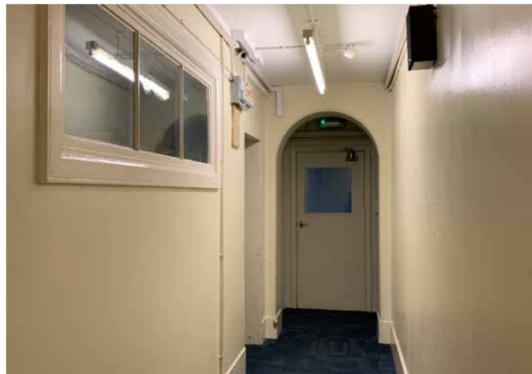
Figure 4.22 Historic arches located at either end of the rear corridor, located behind the chapel at second-floor level, provide a source of interest to the building
