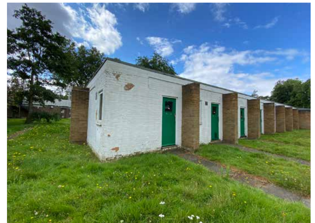
Figure 4.32 Typical late-twentieth century ancillary buildings dispersed throughout the Site
