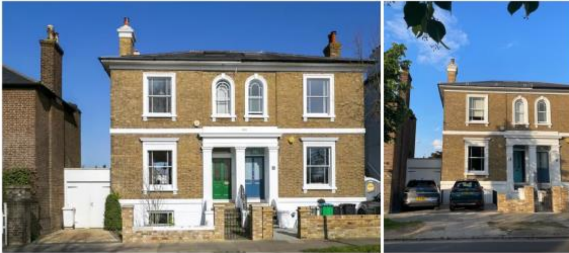
Fig 1. Site prior to / after the removal of the front boundary wall
