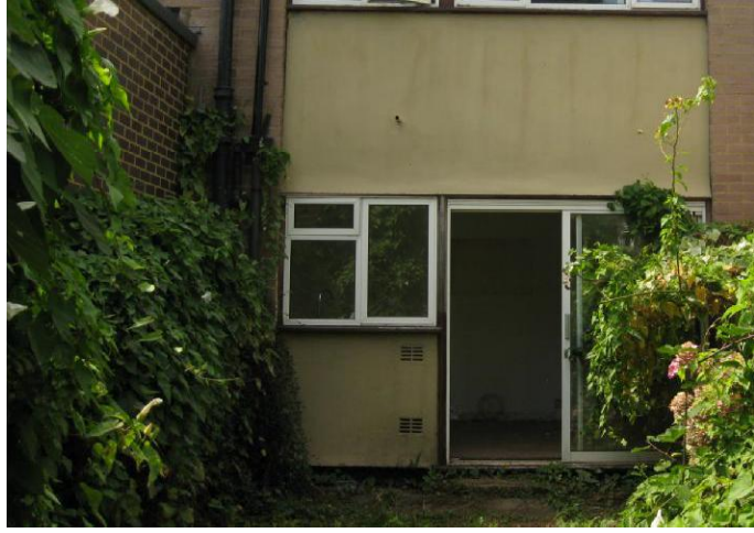
REAR OF 9 RICHMOND ROAD
