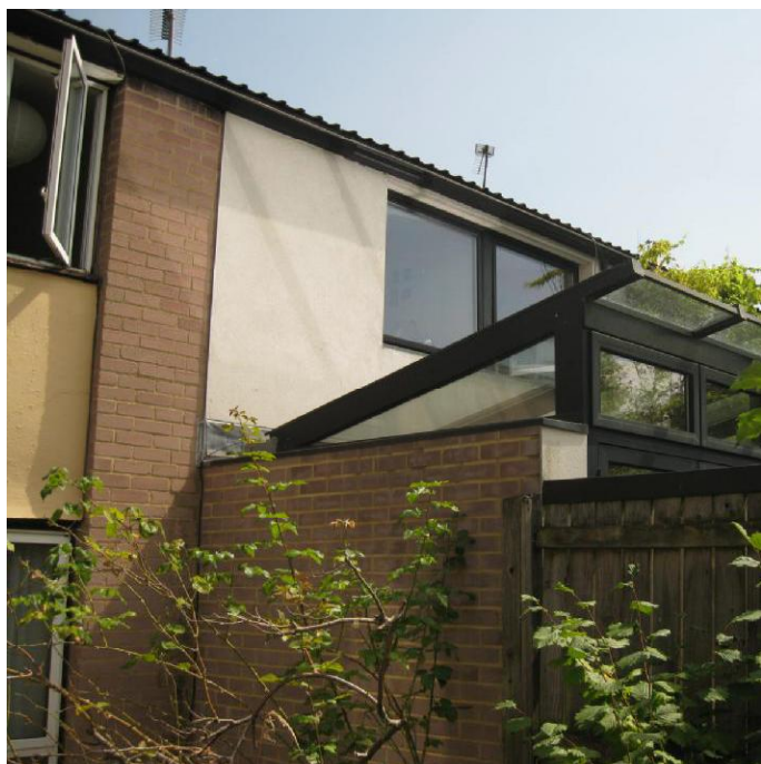
FRONT EXTENSION OF NO. 11
