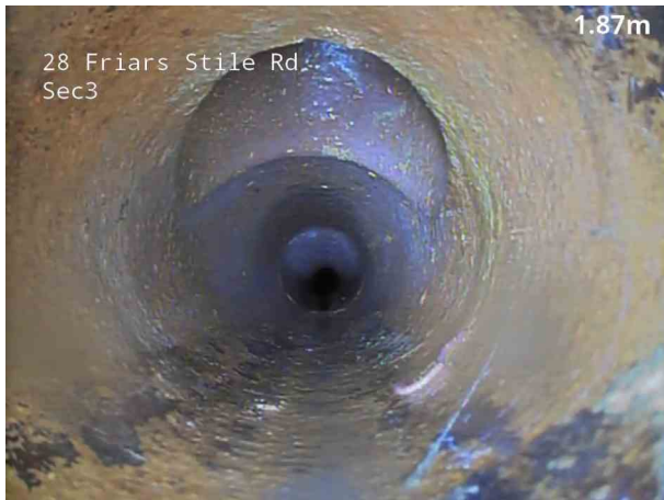
3, 00:01:22, 2.10 m Junction at 12 o'clock, 100mm dia, Serving WC
