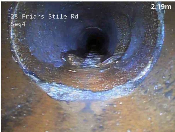
3, 00:00:42, 2.40 m Junction at 3 o'clock, 100mm dia, Serving basement gully.
