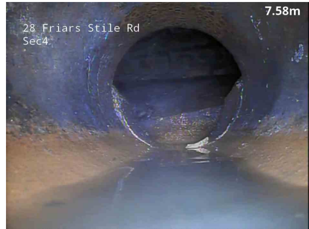
8, 00:02:02, 7.60 m Water level, 5% of the vertical dimension
