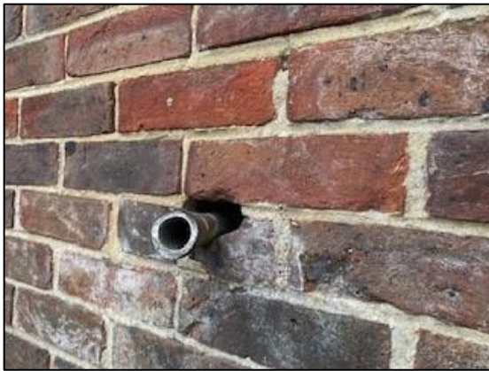
Photograph 17: Building 2 southern aspect.
