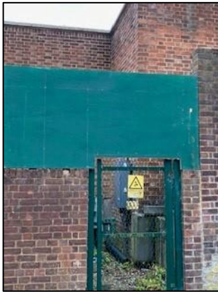
Photograph 15: Building 3 northern aspect.
