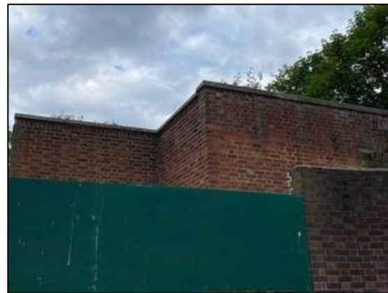
Photograph 14: Building 3 northern aspect.
