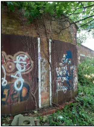
Photograph 9: Building 1 eastern aspect.
