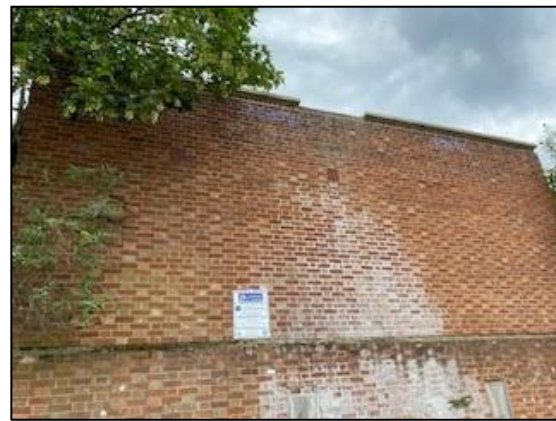
Photograph 12: Building 1 northern aspect.
