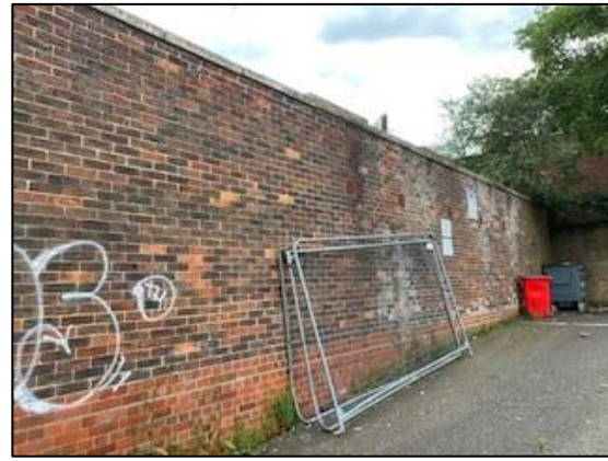
Photograph 16: Building 3 eastern aspect.
