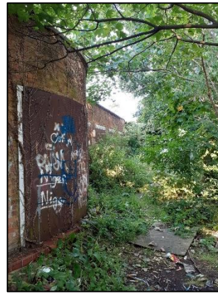
Photograph 10: Building 1 eastern aspect.
