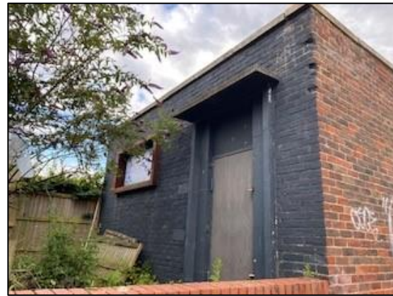
Photograph 18: Building 4 southern aspect.
