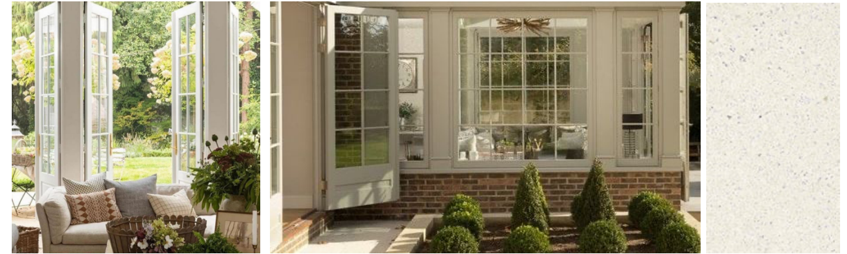
French doors to the garden room extension with brick detailing under the windows to the side. White render to walls.
