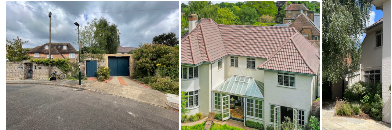
Photo 1-Front gates face the road, with original arch gate to no.15 visible on the left. Photo 2- recent reroofing of no.17 with concrete pantiles to the house and rear conservatory infill (1990) Photo 3 - lean to porch to front elevation.
