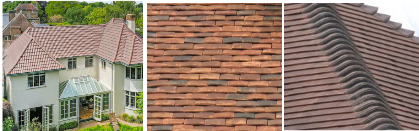
Existing concrete pantile. Proposed clay tiles - mix of reds, medium and dark clay tiles. Example granny bonnet hip detail.
