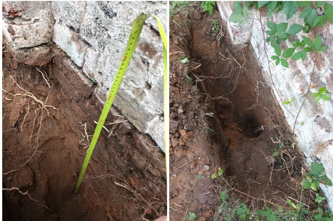
Photograph 1 – Founding Depth (1m)
