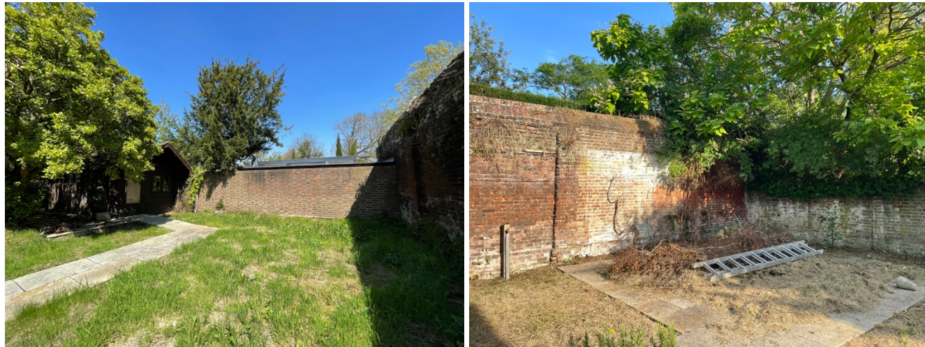
View to the boundary no. 15 with outbuilding beyond.
