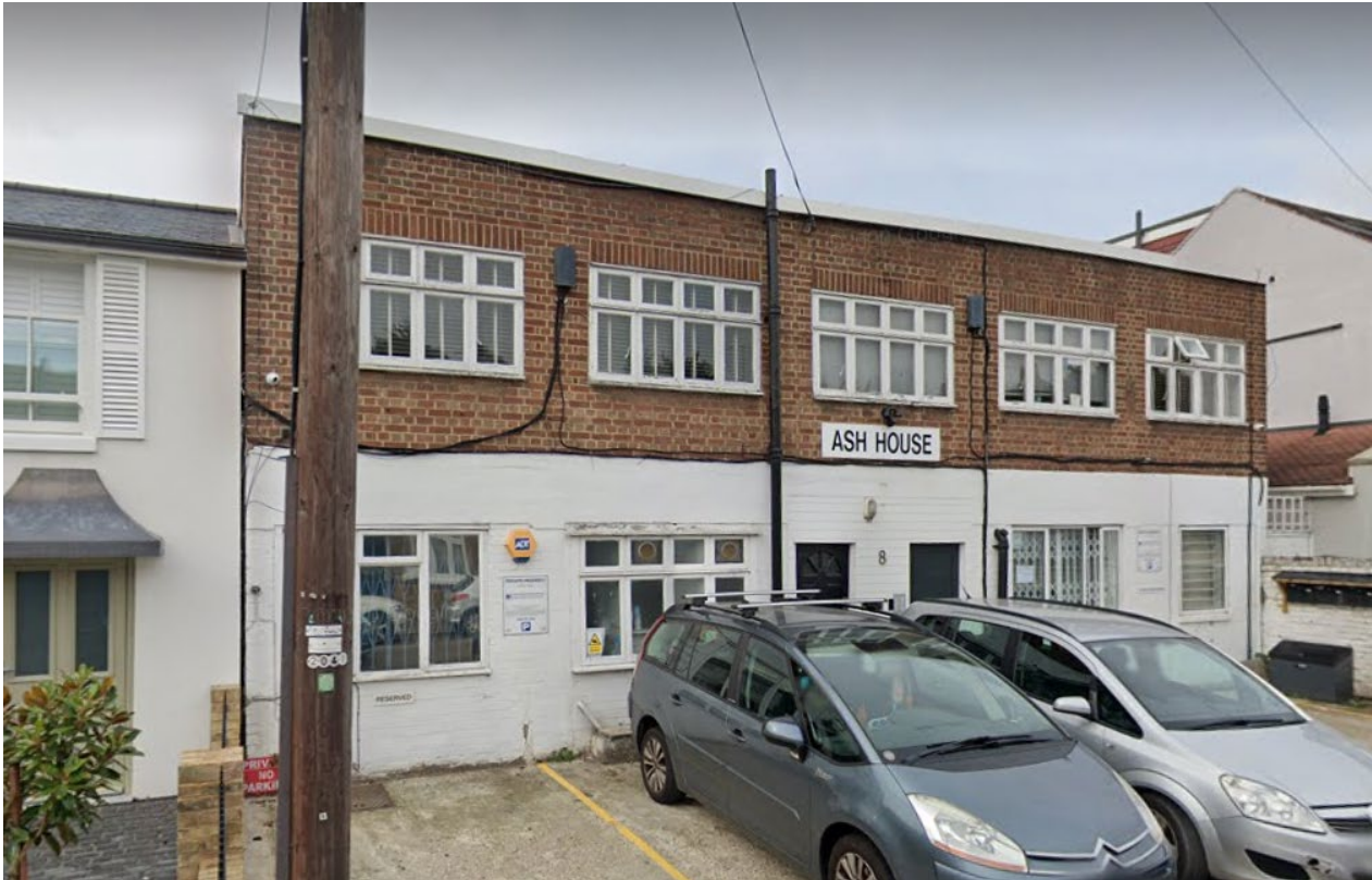
Figure: Existing Building (showing detached nature)
