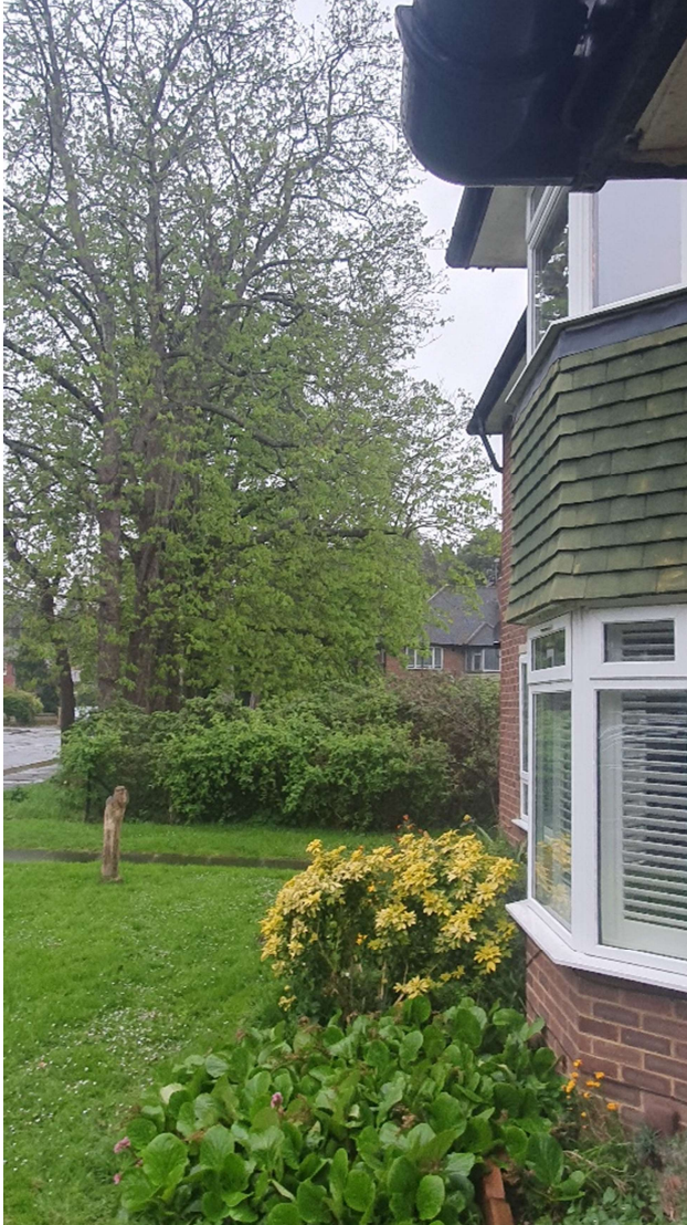
Figure 7: The edge of the tree canopy viewed along the front facade of 34 Cambridge Park from the east. March 2024
