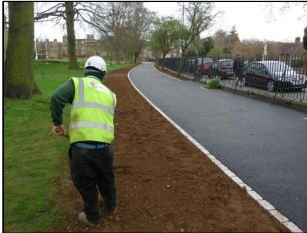
Fig 14 – All 'making good' topsoil will be BS3882 compliant and raked out by hand to no greater depth than 100mm.
