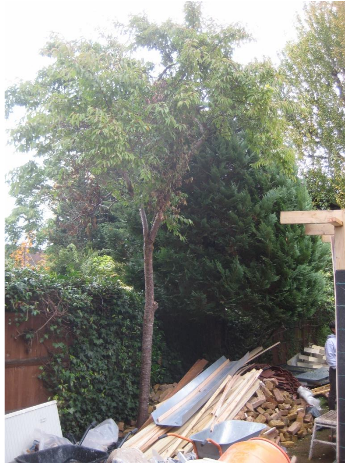
Image 1 – T1 & T2 – Existing materials to be removed carefully by hand before tree protection is installed.
