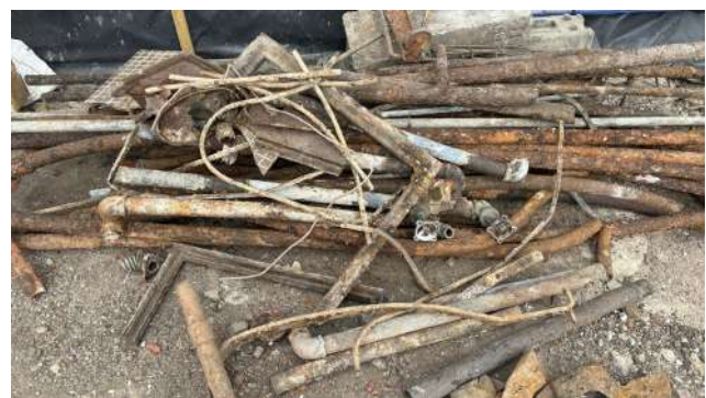
Photo Four: Fuel supply pipeworks 'chased out' and removed.
