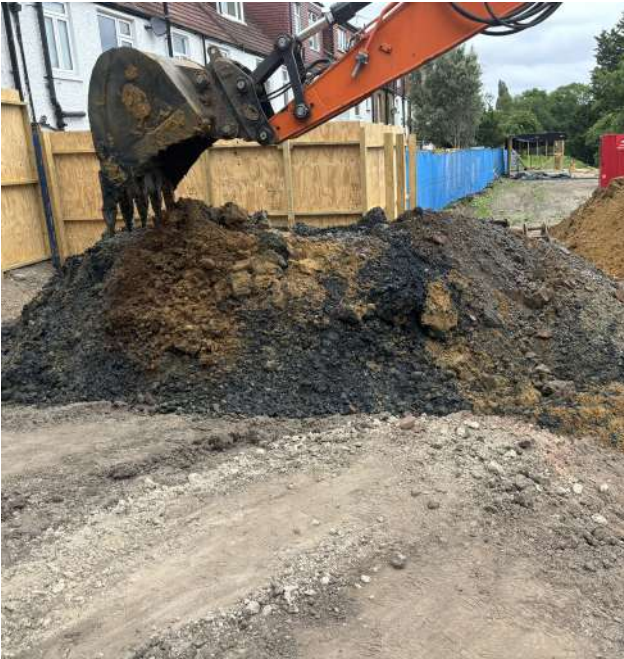
Photos Eleven: Stockpiling of hydrocarbon impacted soils (subsequently removed from site).
