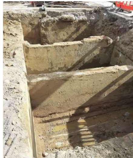
Photo Two: Tank bund, once fuel tanks had been removed.
