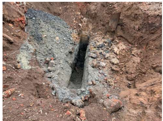
Photo Eight: The sand and gravel layer, underlying the clay, showed dark staining and had a pronounced hydrocarbon odour.
