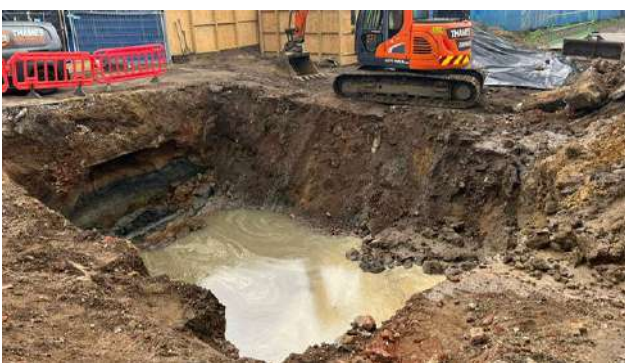
Photo Three: Excavation once tanks/bund and adjacent interceptor had been removed.
