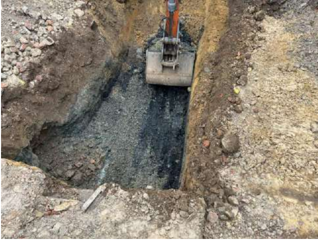
Photos Nine and Ten: Progression of remedial excavation in area of former tanks
