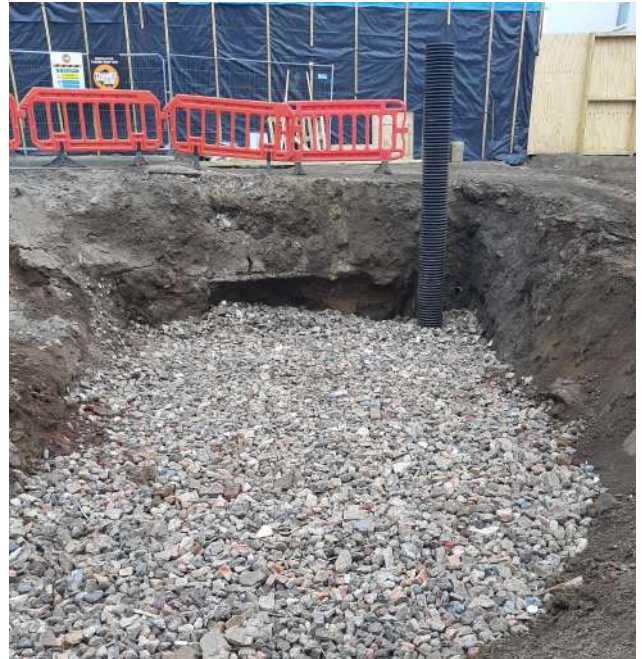
Photo Twelve: The remedial excavation partially backfilled.
