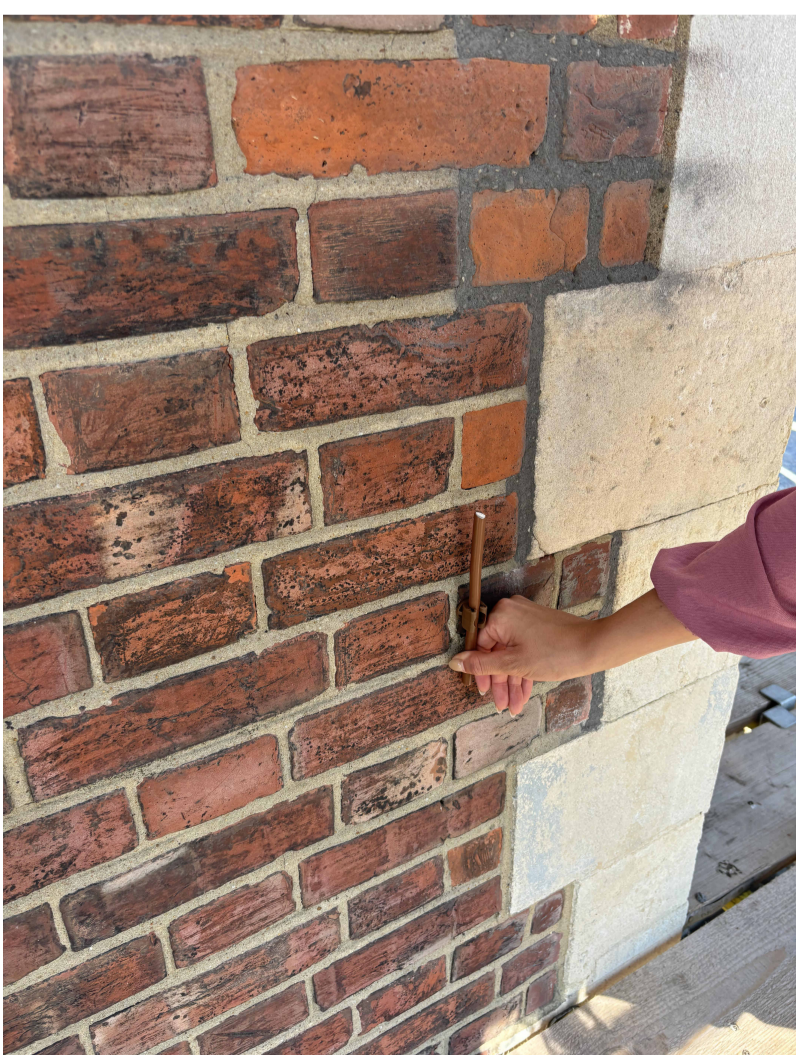
Image 1 Thin copper Lightning Protection tubes dropped down on elevations as per locations on drawing above
