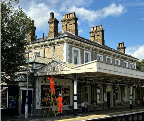
Image 12 – Teddington Station Rear Elevation viewed from South East
