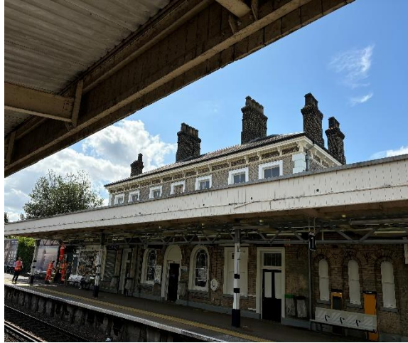
Image 13– Teddington Station Rear Elevation viewed from North West
