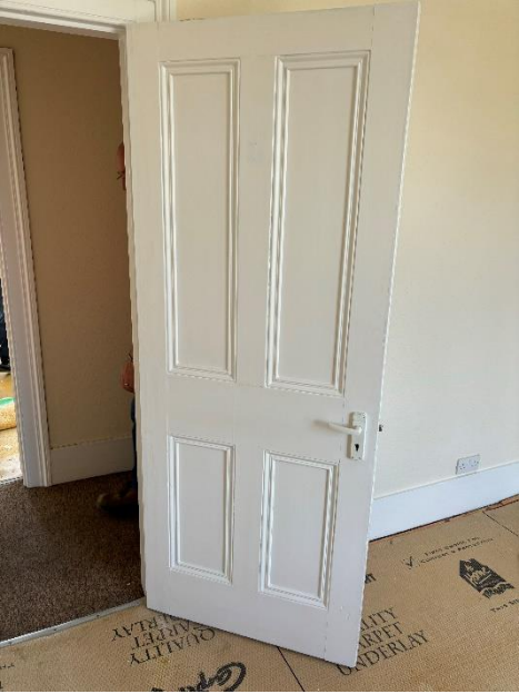
Image 9 – Typical First Floor Four Panel Door
