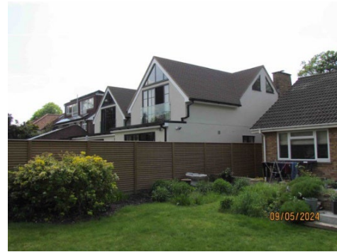
Tanglewood, Marlborough Road – rear extension
