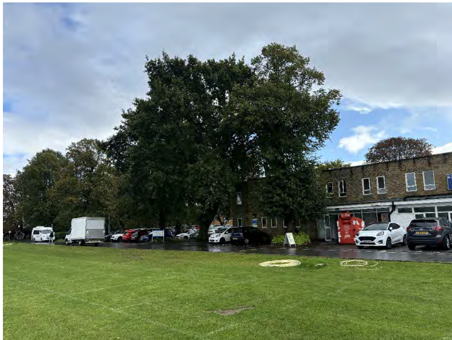
Figure 1: View of T1, looking southeast
