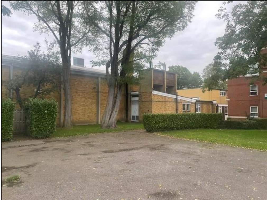
Plate 7: View looking NE, towards the W and S sides of the site from the courtyard to the S of R Block.
