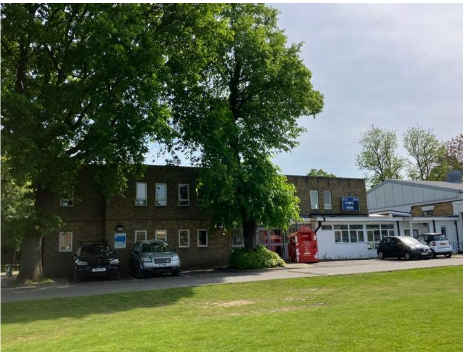
Figure 3 – Photo of the existing teaching block to be redeveloped
