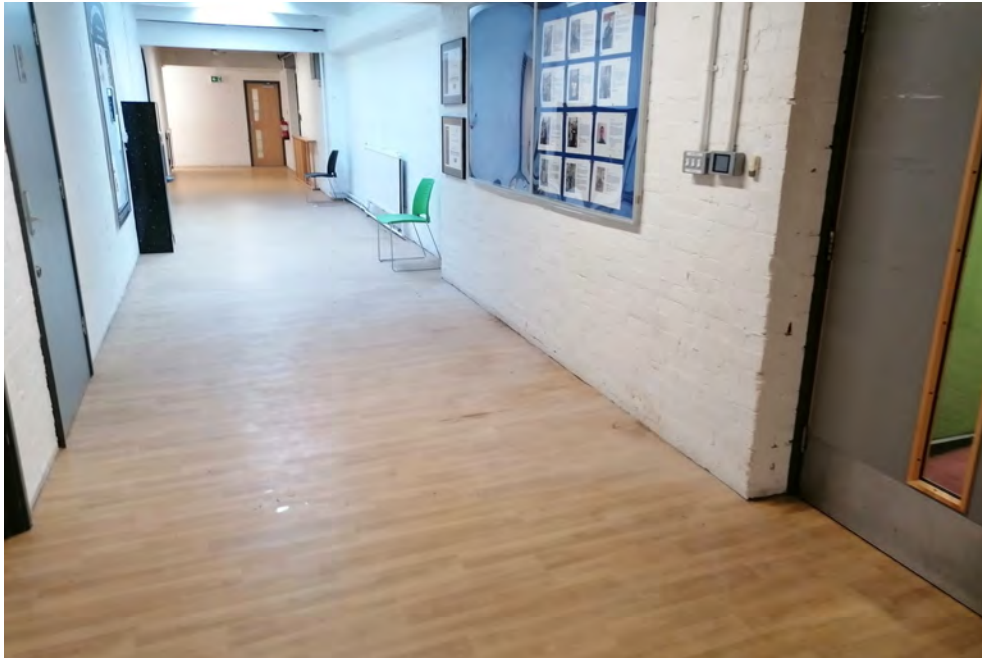
Situated internally at location FTP03 showing corridor.
