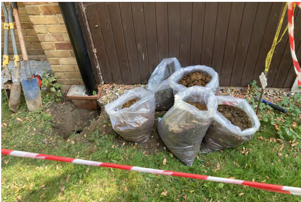
Photo of FTP01 arisings
