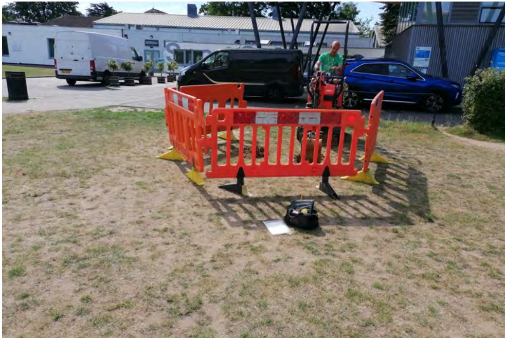
Situated externally, north of the subject building facing south showing the sports pitch and location SA02
