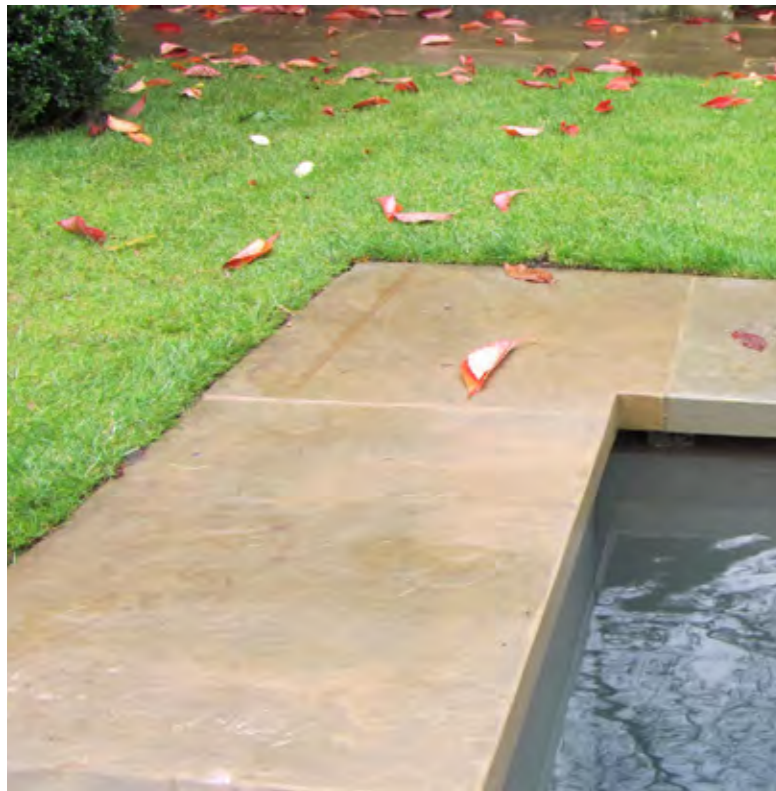
Reclaimed York stone pool coping
