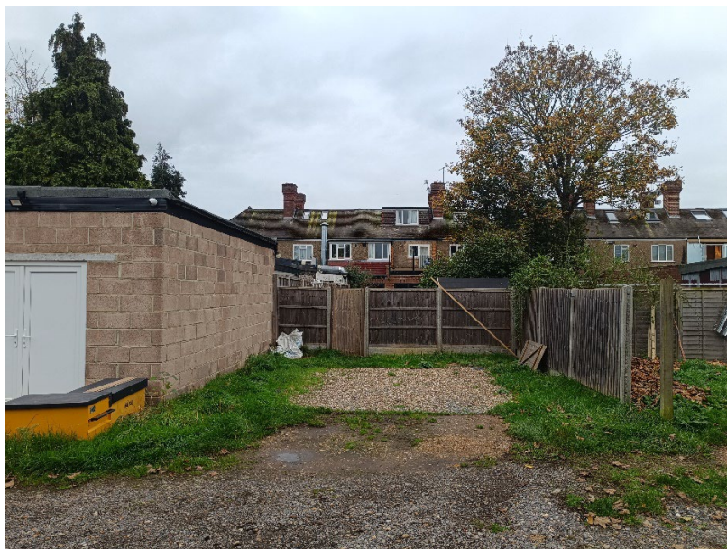
Image 2: Location of proposed outbuilding (Source: site visit 29 October 2024)
