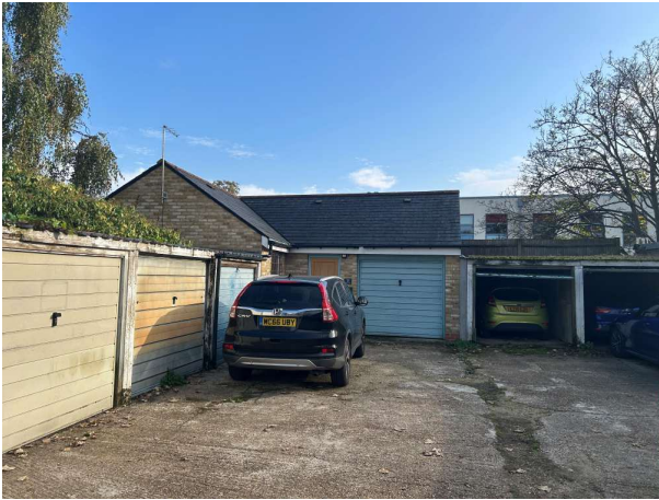
South Facing Elevation From Garage Forecourt
