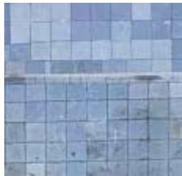
Area of new paving using reclaimed or matching existing concrete paving
