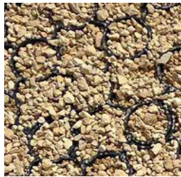
Car parking bays: Reinforced Gravel (permeable)
