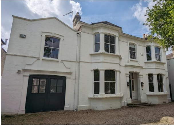
Figure 7. Principle (north) elevation viewed from the front garden
