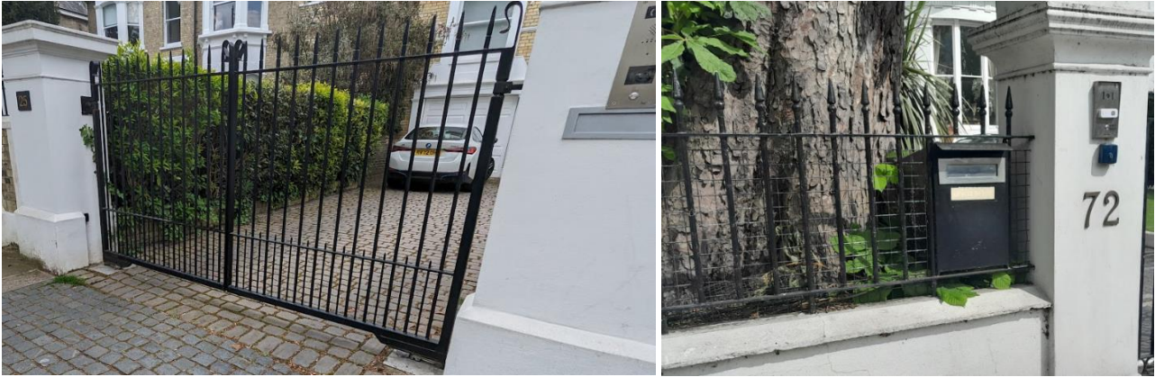
Figure 12. Gates to no.25 (left), and characteristic railings above the low boundary wall of no.72 opposite (right)
