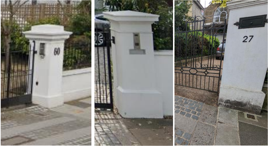
Figure 11: Example of intercoms and integrated letterboxes on Lonsdale Road
