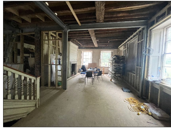
Photo of elevation B
