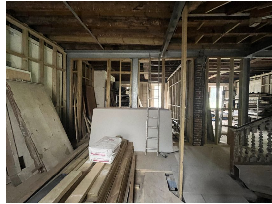
Photo of elevation B
