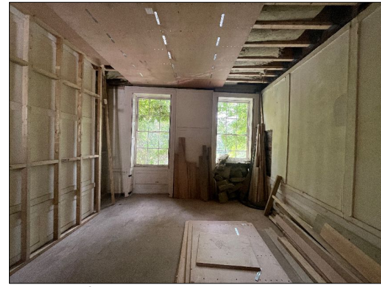
Photo of elevation B
