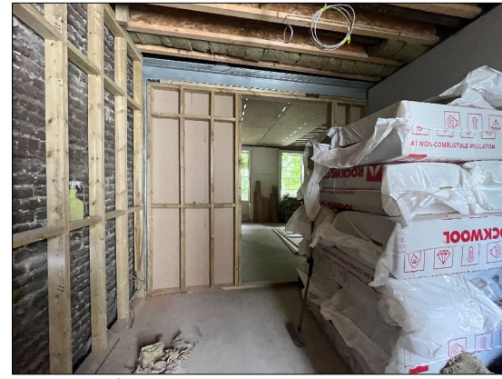
Photo of elevation B
