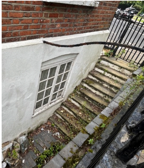
Figure 25: Flight of steps to the front lightwell to basement
