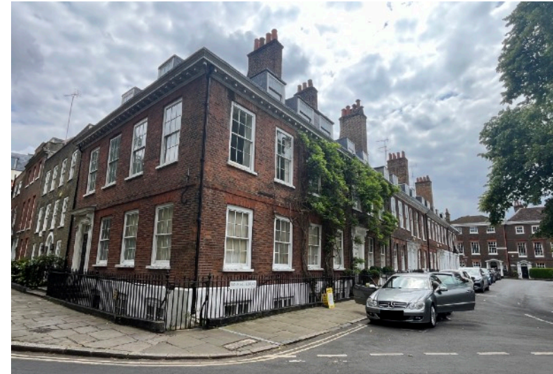
Figure 3: No 32 The Green viewed from the North at the corner of The Green and Old Palace Terrace. Photograph taken June 2024
