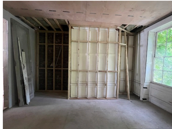
Figure 9: Room F1 showing load bearing stud work in front of a
