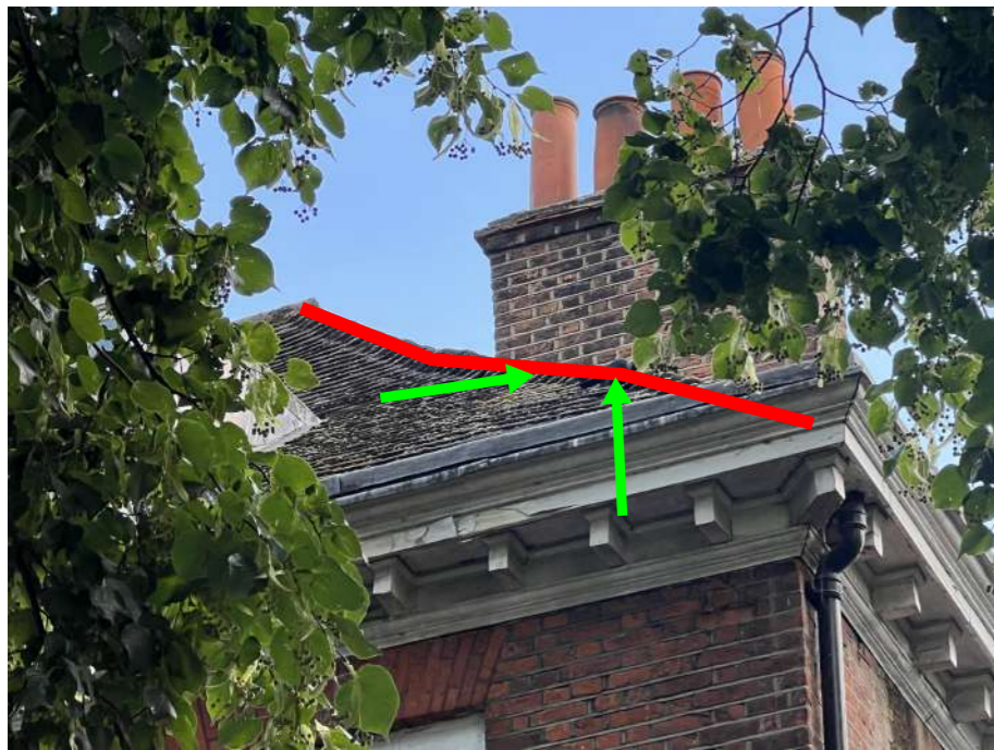
Deflected shape of HIP and interior supports
