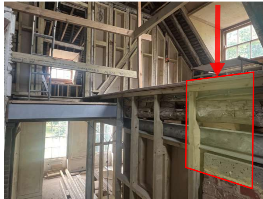
The stair wall immediately below where support is required.
