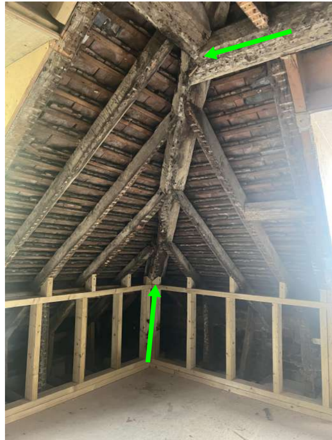
Interior view of sidewall support (vertical) and purlin prop (horizontal)
