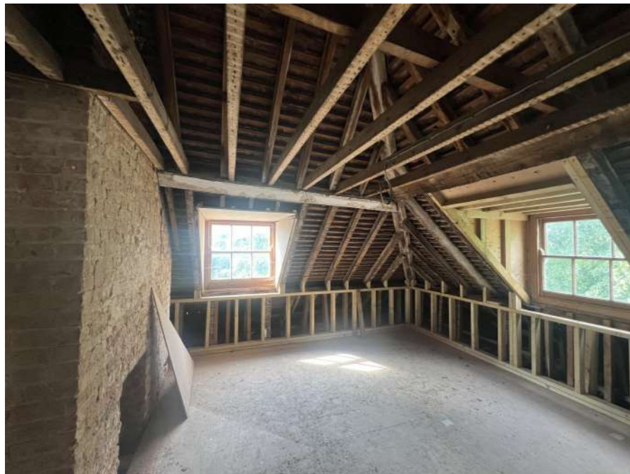
Interior view of sidewall support (vertical) and purlin prop (horizontal)
