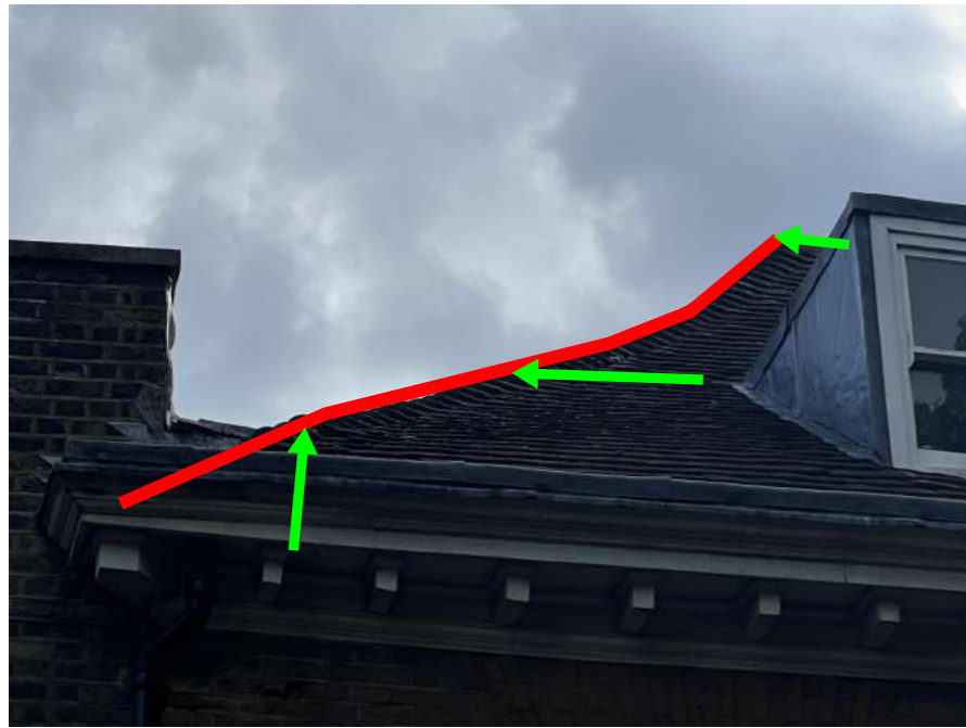
Deflected shape of HIP and interior supports
