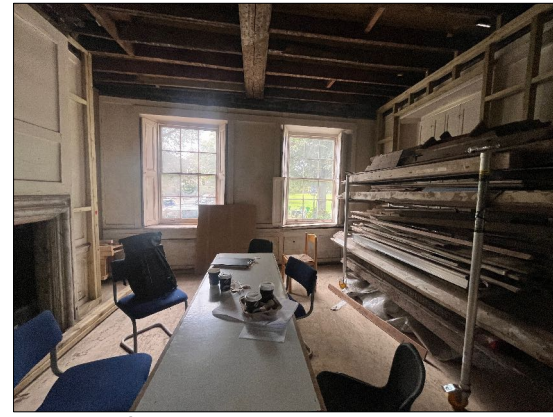
Photo of elevation B
